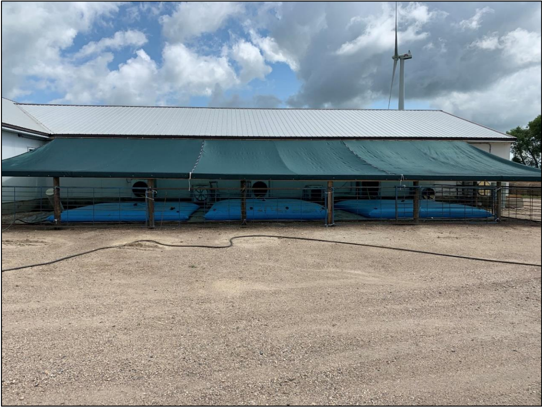
Figure 4.1. Photo of filled water bladders under a lean-to shelter (North side)
