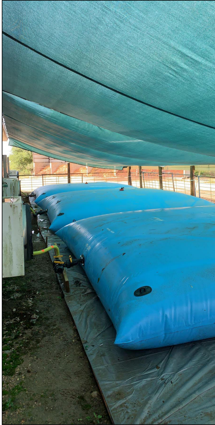
Figure 4.3. Photo of full water bladders and pump connections (East side)
