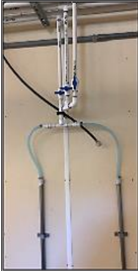
Figure 4.4. Photo of water system and manifold from ceiling to standpipe
