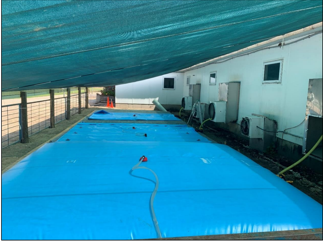
Figure 4.2. Photo of full (foreground) and empty water bladders (West side)
