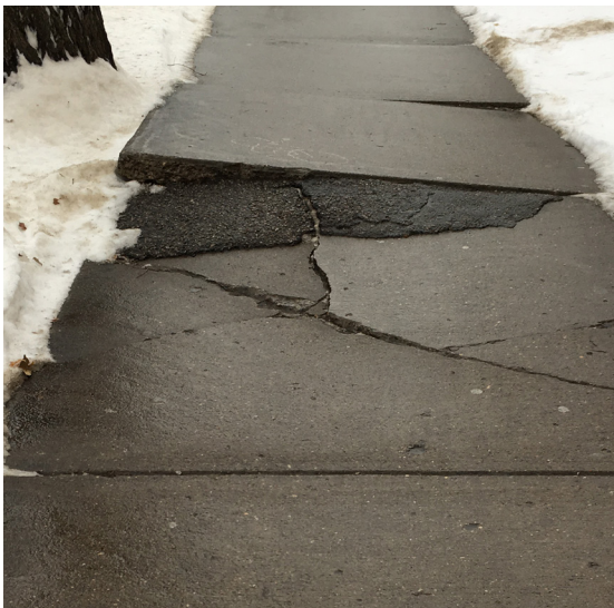
FIGURE 28 : HEAVING AND CRACKING PANELS
