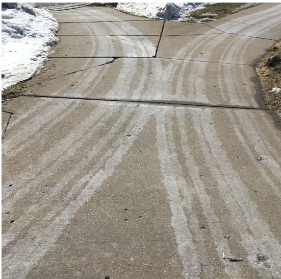
FIGURE 4 : SIDEWALK SURFACE TRACES - SALT BRINE STREAKS
