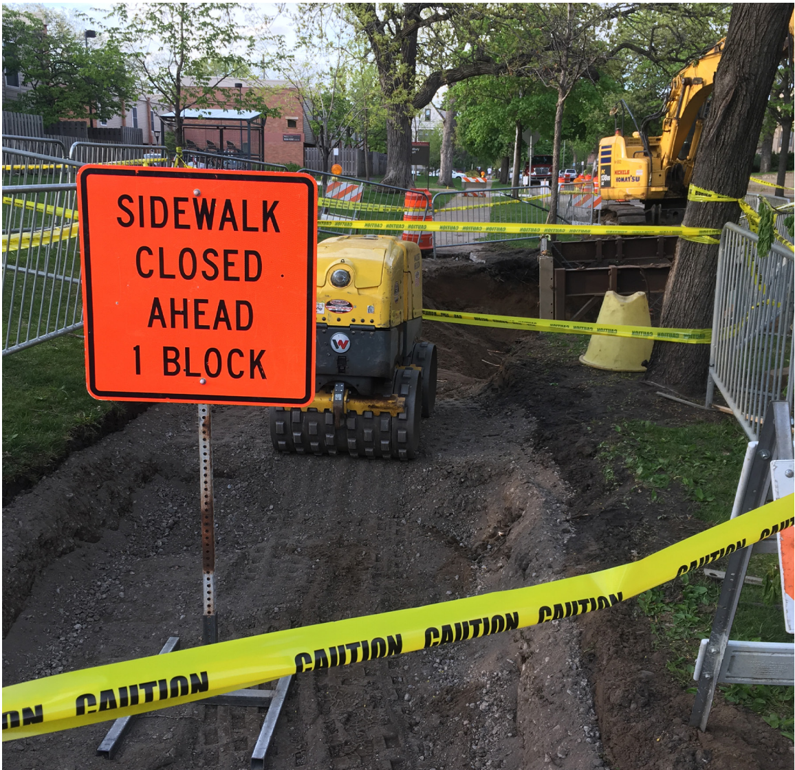
FIGURE 29 : COMPACTED AGGREGATE, COMPACTED SOIL, TRENCH ROLLER (COMPACTOR) 108
