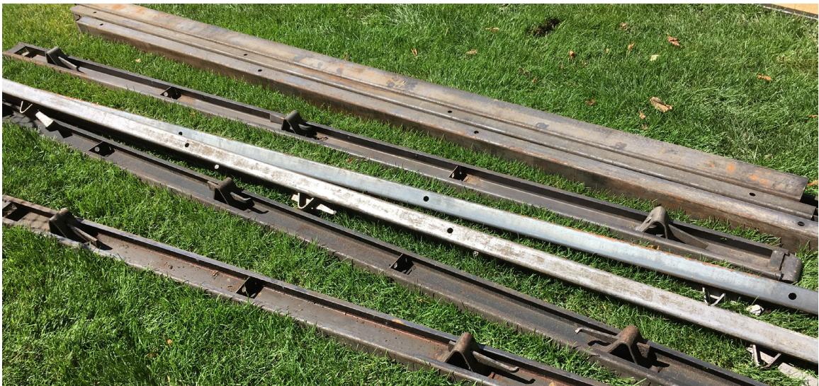
FIGURE 15 : LAYING THE FORMS
