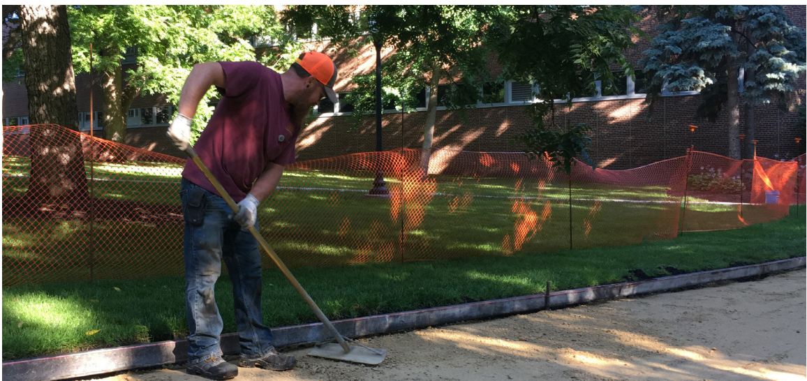
FIGURE 14 : PREPPING THE SITE
