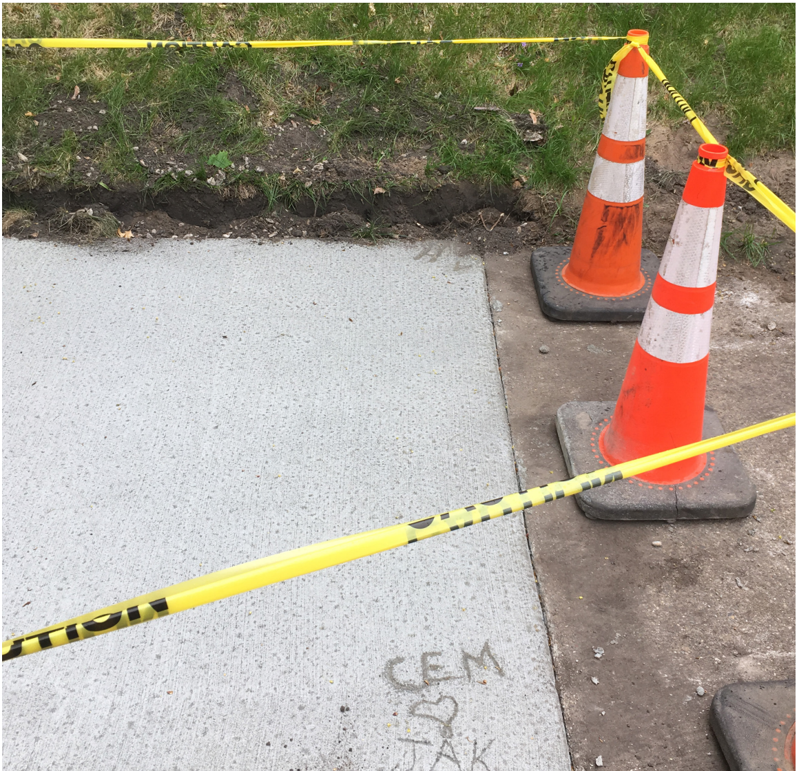
FIGURE 31 : TREE ARCH, ASPHALT RAMP, REPLACEMENT PANEL
