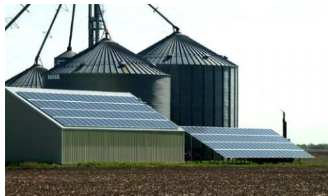
Solar exceeds expectations at Guentzel Family Farms in Eagle Lake
