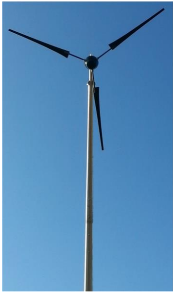
Two 10 kW Wind Turbines
