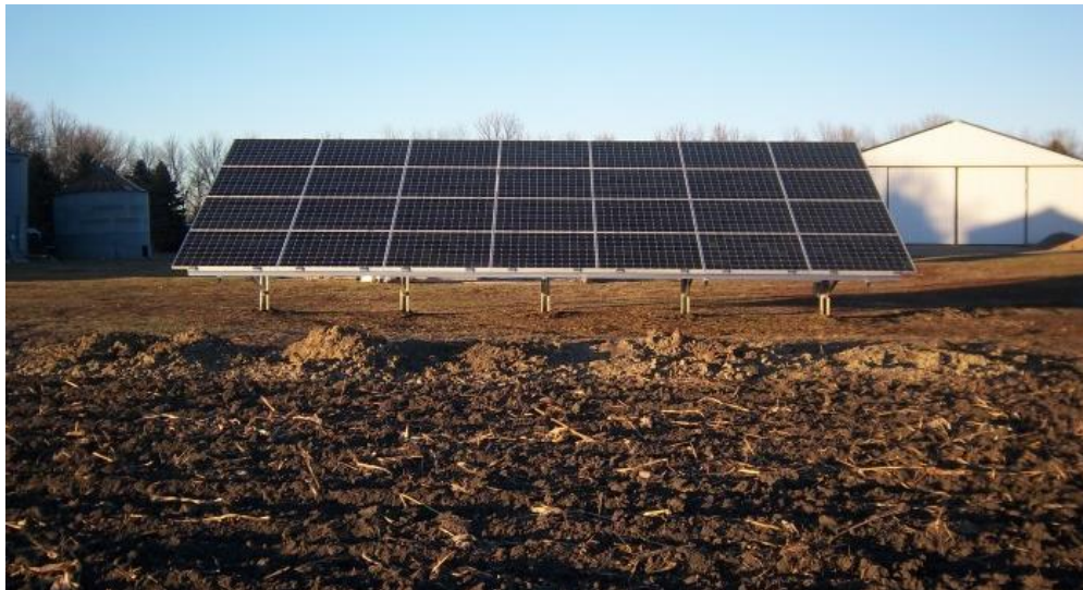
Photo Credit: Green Energy Products
