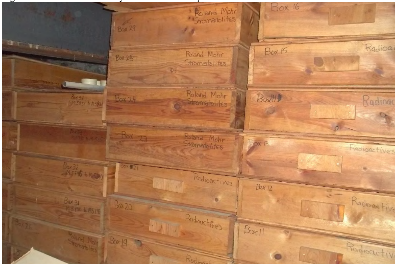
Figure 2.2 State of the Pillsbury Hall subbasement prior to abatement
