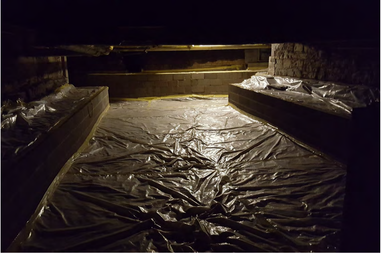
Figure 2.3 State of the Pillsbury Hall subbasement after abatement
