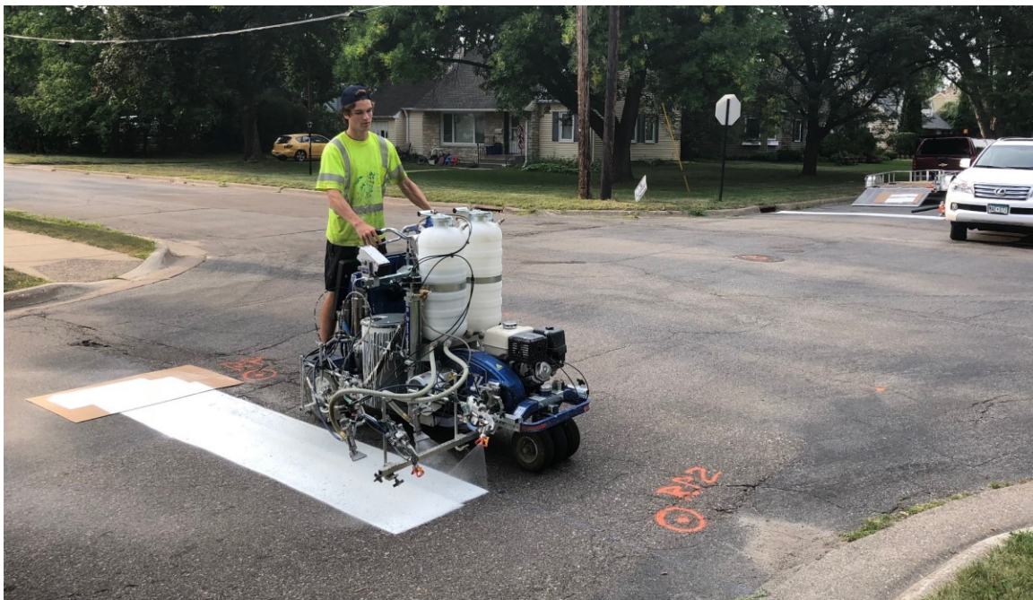
Figure 3.3 Painting of stop lines
