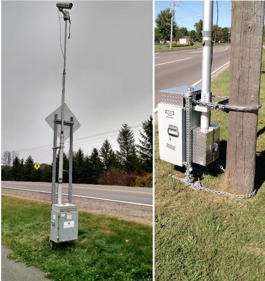
Figure 3.2 MTO camera systems braced on sign post (left) and utility pole (right)
