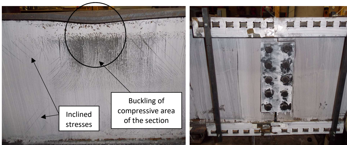
(a) Failure of the beam at center span
