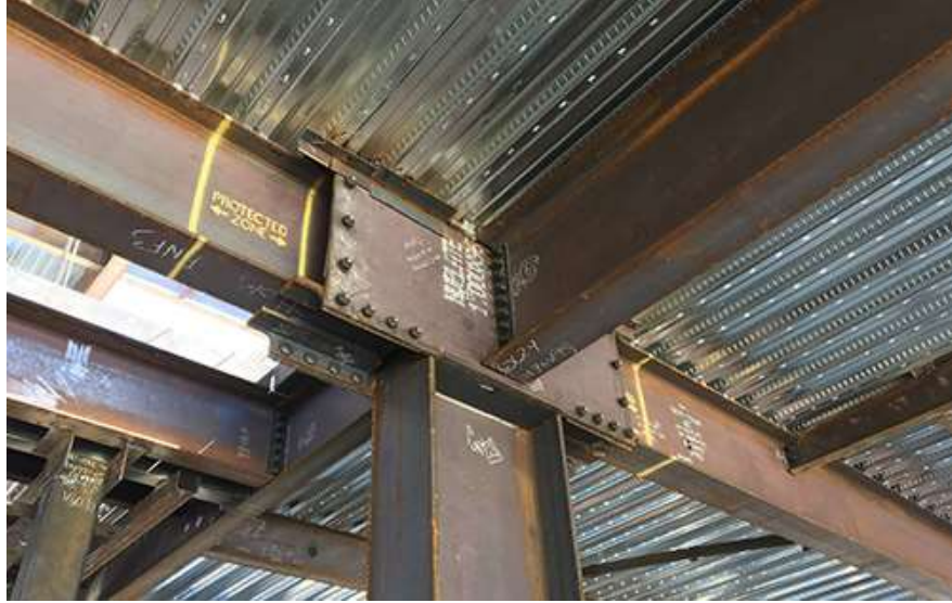
Fig. 1-6 SidePlate® connection implemented in a steel frame [16]
