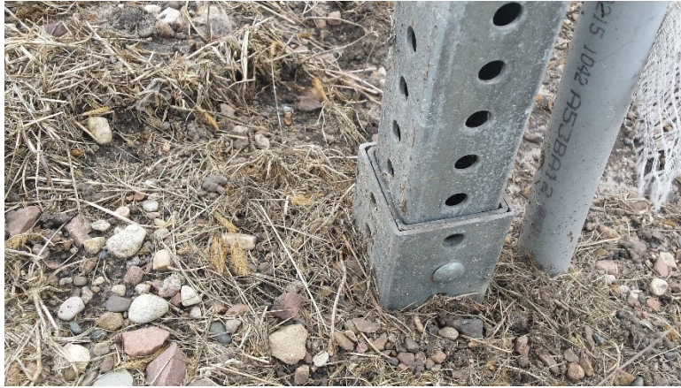
Figure 8.5 – Image of breakaway base connection for RICWS
