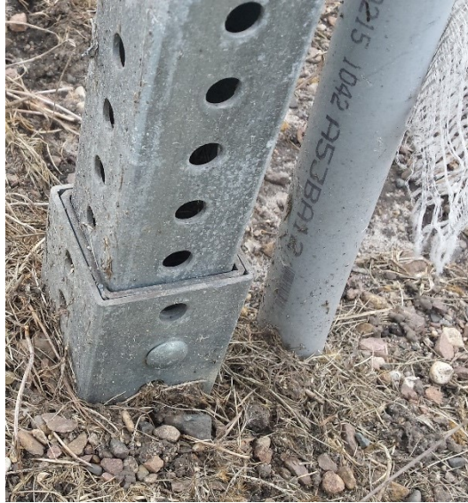
Figure 2.6 – Example of RICWS breakaway connection
