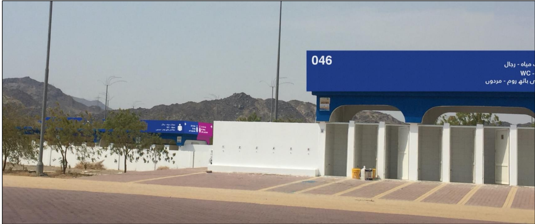
Image 17: WC signs on buildings that serves both genders
