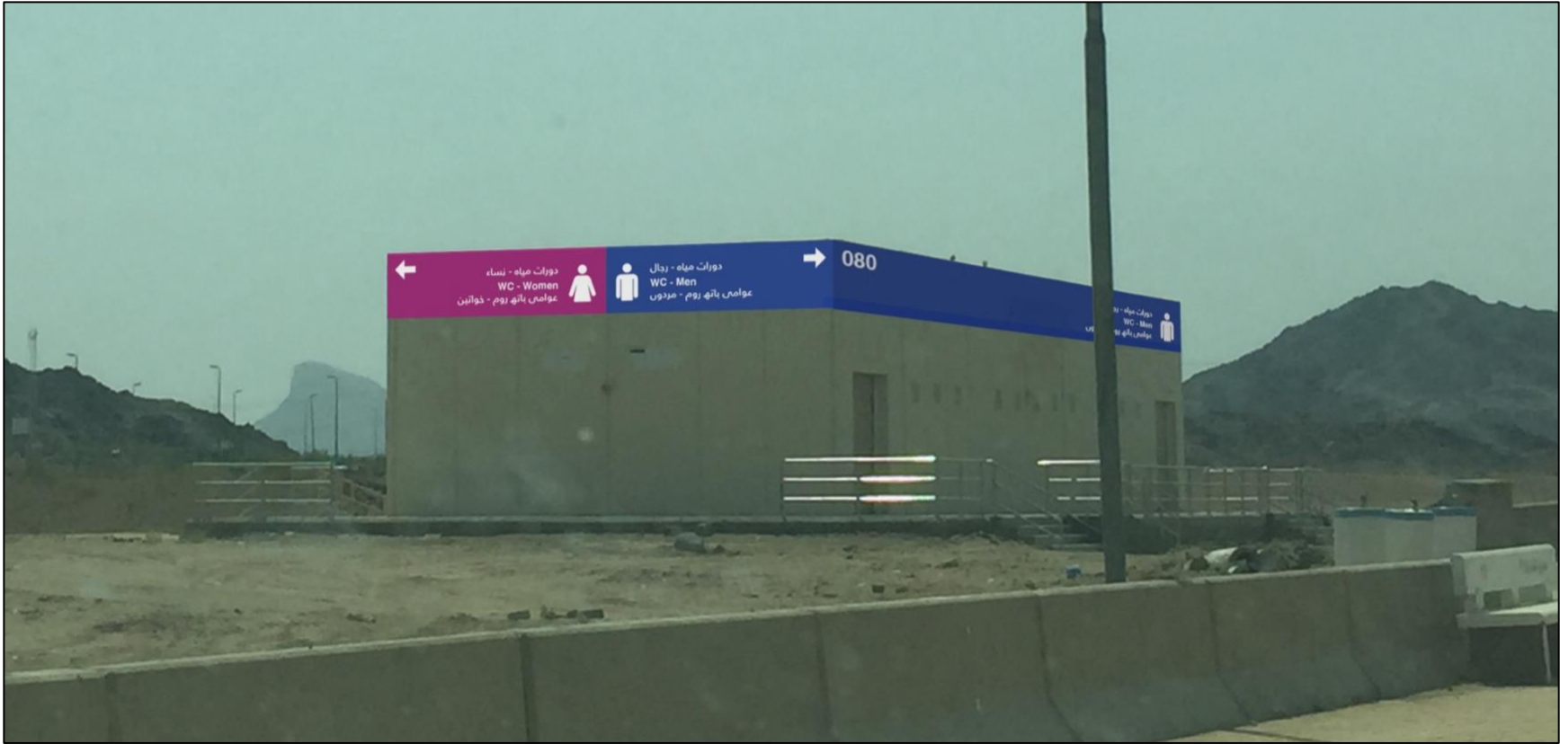
Image 16: WC signs on buildings that serves both genders
