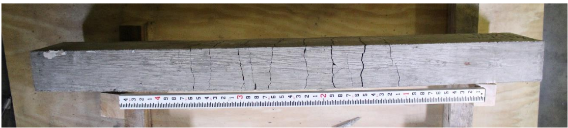
Figure D.87. Mixture 10 (10UV10FA2) beam #20: concrete beam bottom view.
