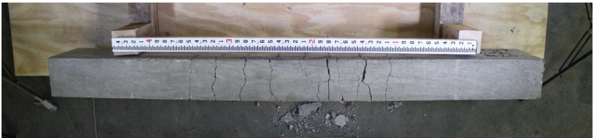
Figure D.15. Mixture 2 (20FA1) beam #20: concrete beam bottom view.
