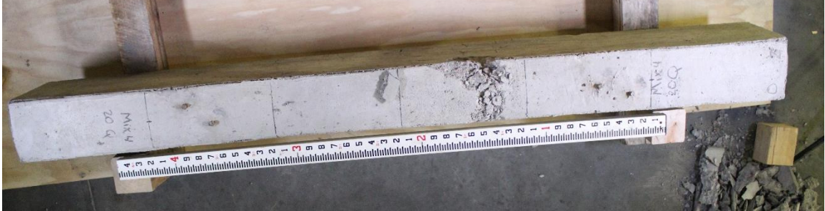
Figure D.31. Mixture 4 (20Q) beam #20: concrete beam top view.
