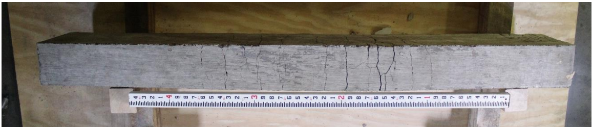
Figure D.78. Mixture 9 (20UV) beam #20: concrete beam bottom view.
