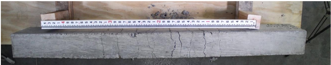
Figure D.54. Mixture 6 (10W10FA2) beam #30: concrete beam bottom view.
