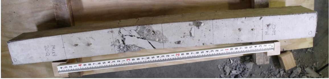
Figure D.34. Mixture 4 (20Q) beam #30: concrete beam top view.
