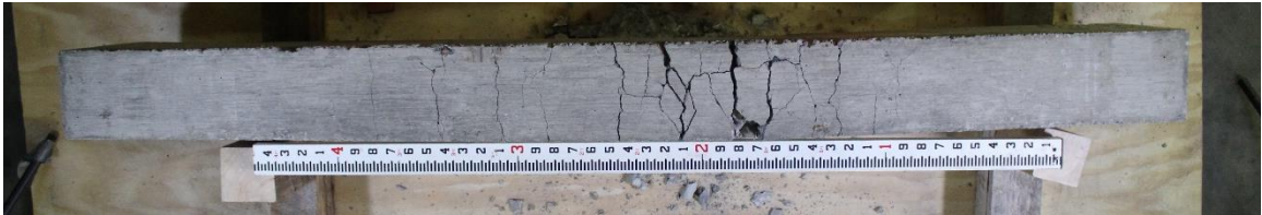
Figure D.48. Mixture 6 (10W10FA2) beam #1R: concrete beam bottom view.
