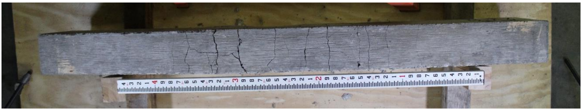
Figure D.57. Mixture 7 (20W) beam #1R: concrete beam bottom view.
