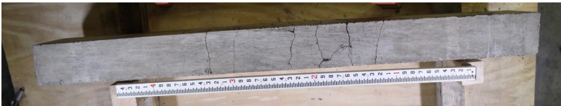
Figure D.21. Mixture 3 (20FA2) beam #1R: concrete beam bottom view.
