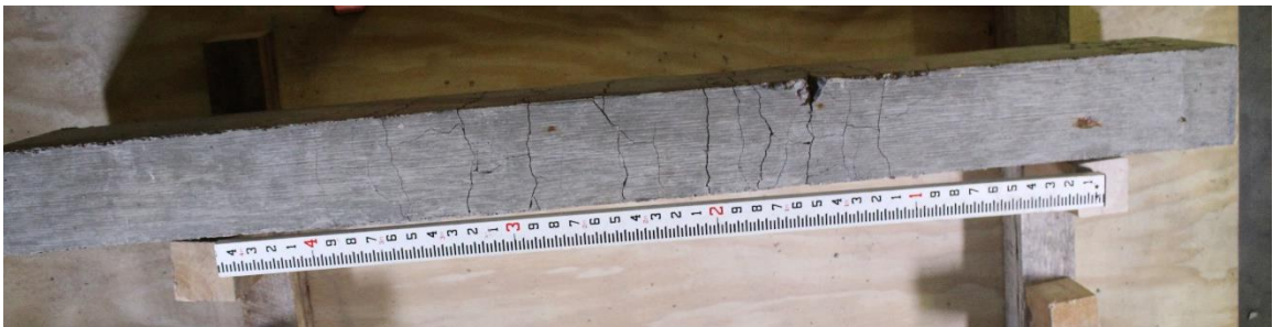
Figure D.66. Mixture 8 (10W10FA1) beam #1R: concrete beam bottom view.
