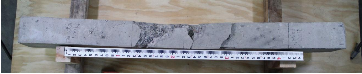
Figure D.1. Mixture 1 (100PC) beam #1R: concrete beam top view.
