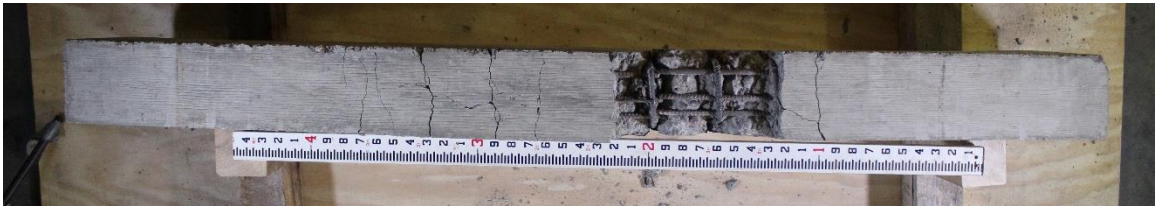
Figure D.51. Mixture 6 (10W10FA2) beam #20: concrete beam bottom view.
