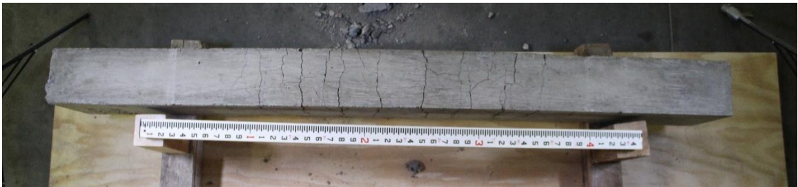
Figure D.12. Mixture 2 (20FA1) beam #1R: concrete beam bottom view.
