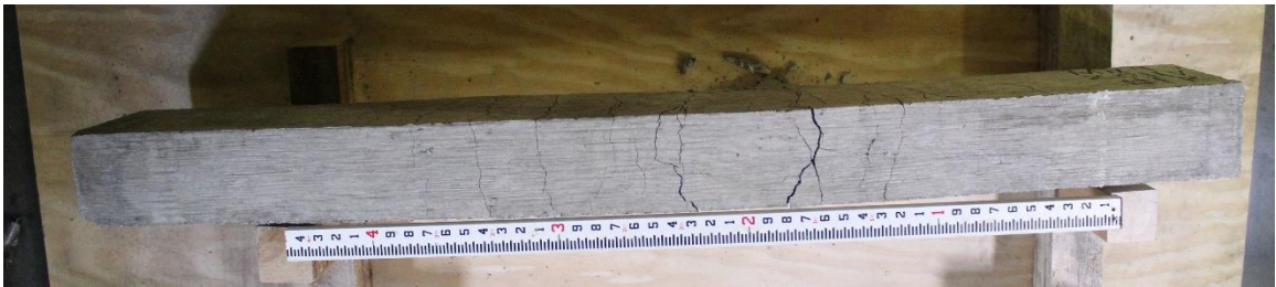
Figure D.75. Mixture 9 (20UV) beam #1R: concrete beam bottom view.
