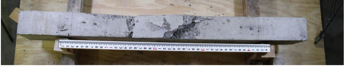
Figure D.4. Mixture 1 (100PC) beam #20: concrete beam top view.
