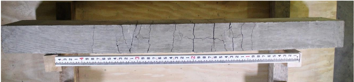
Figure D.72. Mixture 8 (10W10FA1) beam #30: concrete beam bottom view.
