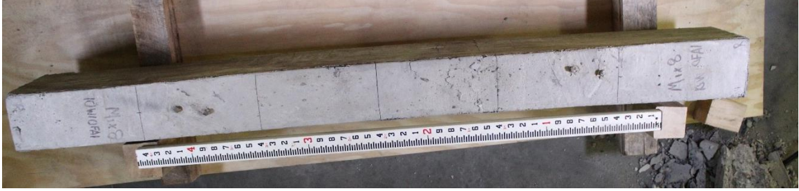
Figure D.64. Mixture 8 (10W10FA1) beam #1R: concrete beam top view.
