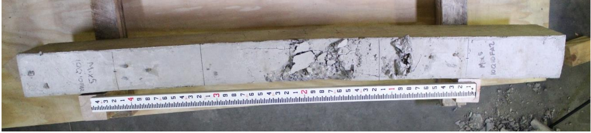
Figure D.40. Mixture 5 (10Q10FA2) beam #20: concrete beam top view.
