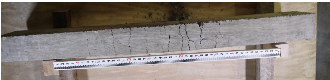
Figure D.27. Mixture 3 (20FA2) beam #30: concrete beam bottom view.
