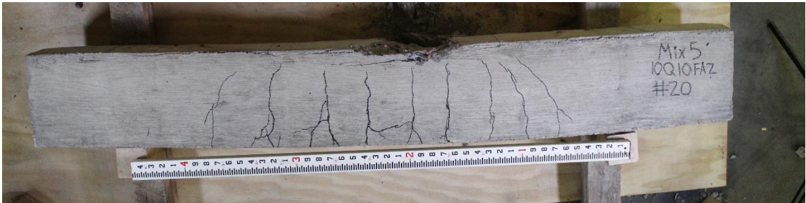
Figure D.41. Mixture 5 (10Q10FA2) beam #20: concrete beam side view.
