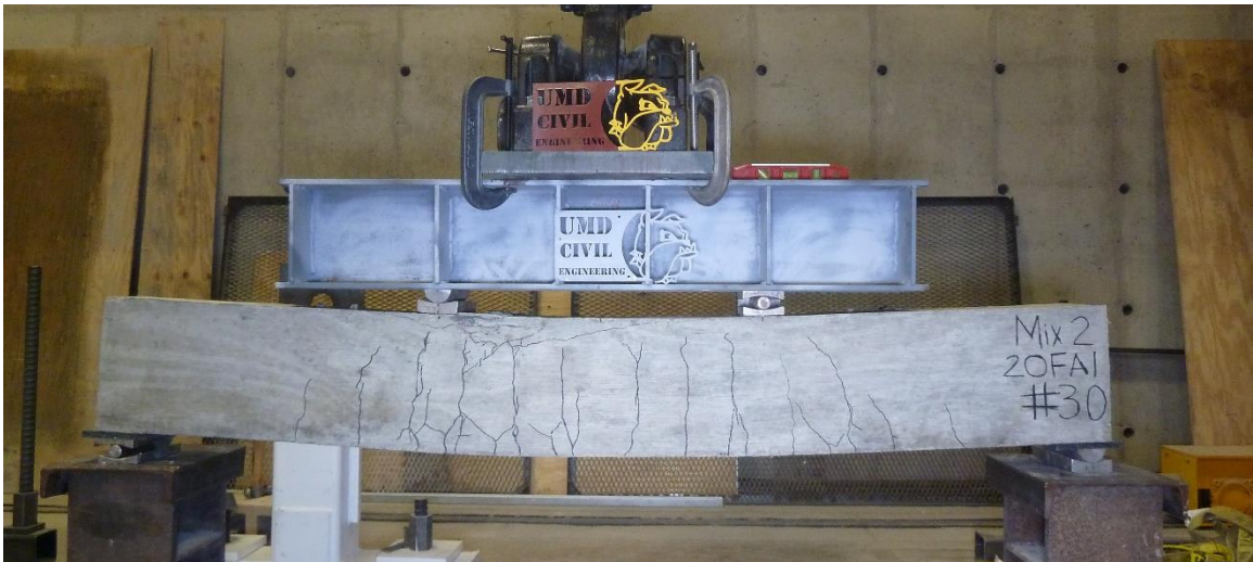
Figure C.12. Mixture 2 (20FA1) beam #30: concrete beam after testing.
