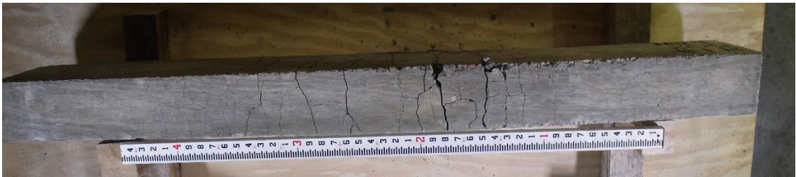
Figure D.30. Mixture 4 (20Q) beam #1R: concrete beam bottom view.
