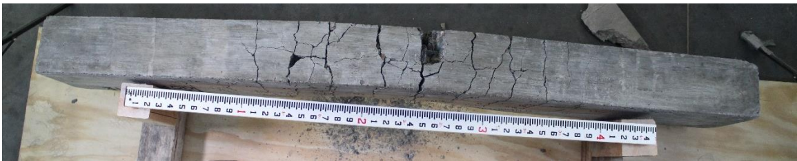
Figure D.3. Mixture 1 (100PC) beam #1R: concrete beam bottom view.
