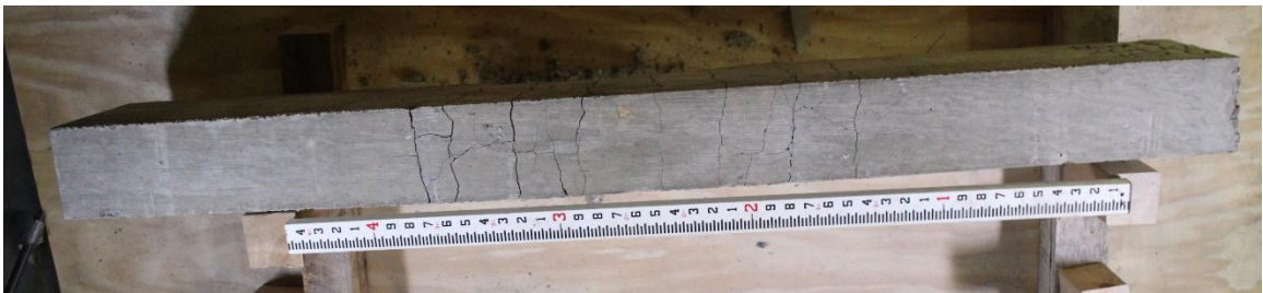
Figure D.24. Mixture 3 (20FA2) beam #20: concrete beam bottom view.
