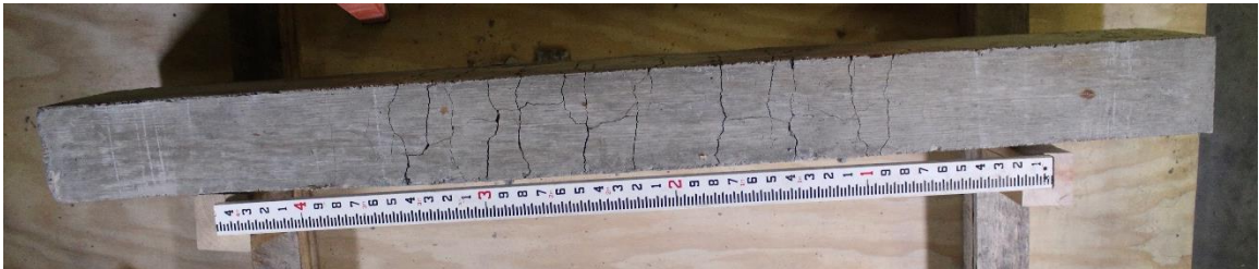
Figure D.18. Mixture 2 (20FA1) beam #30: concrete beam bottom view.
