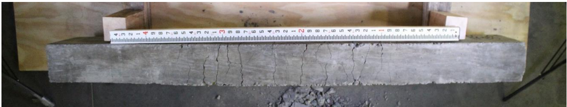
Figure D.9. Mixture 1 (100PC) beam #30: concrete beam bottom view.
