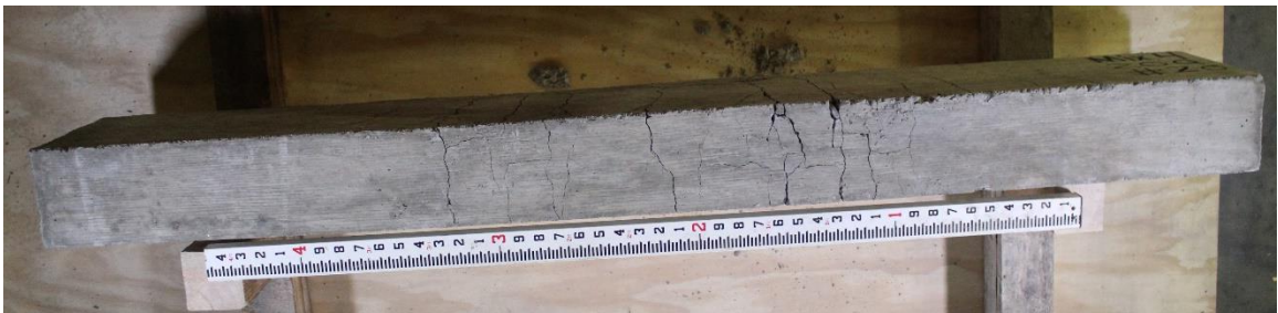
Figure D.33. Mixture 4 (20Q) beam #20: concrete beam bottom view.
