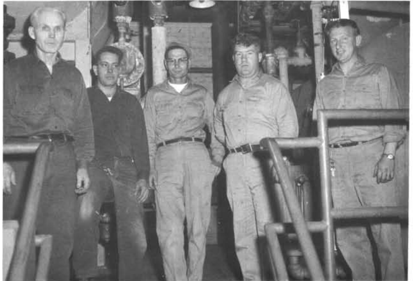
Pictured to the RIGHT are the heating plant employees, William Bohach, Elwood Hill, Felix Baird, Willard Weiss, and Donald Wieland.
