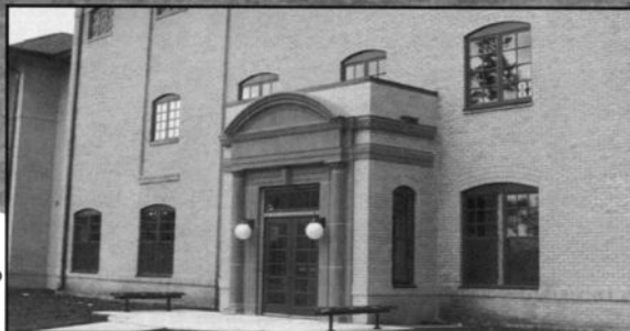
Kiehle Hall Completion Page 22
