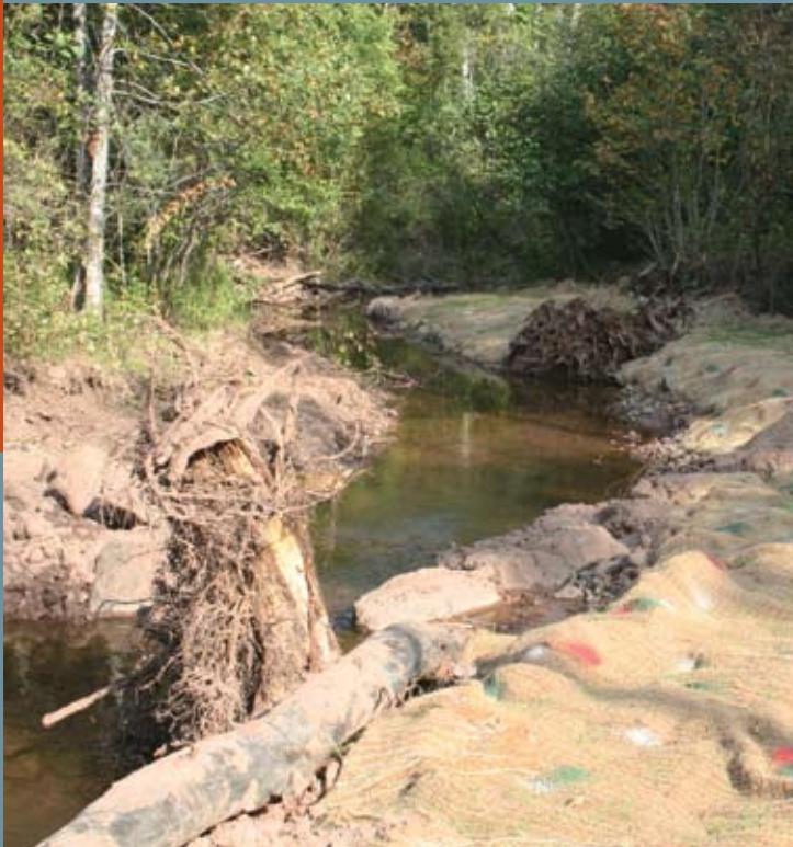
Amity Creek restoration project completed in 2009.
