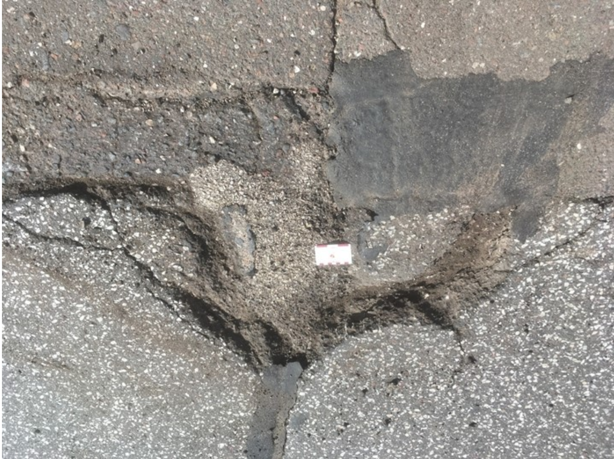
Figure 2.51 Pothole prior to repair: Proctor, MN, field trial site, June 20, 2018.
