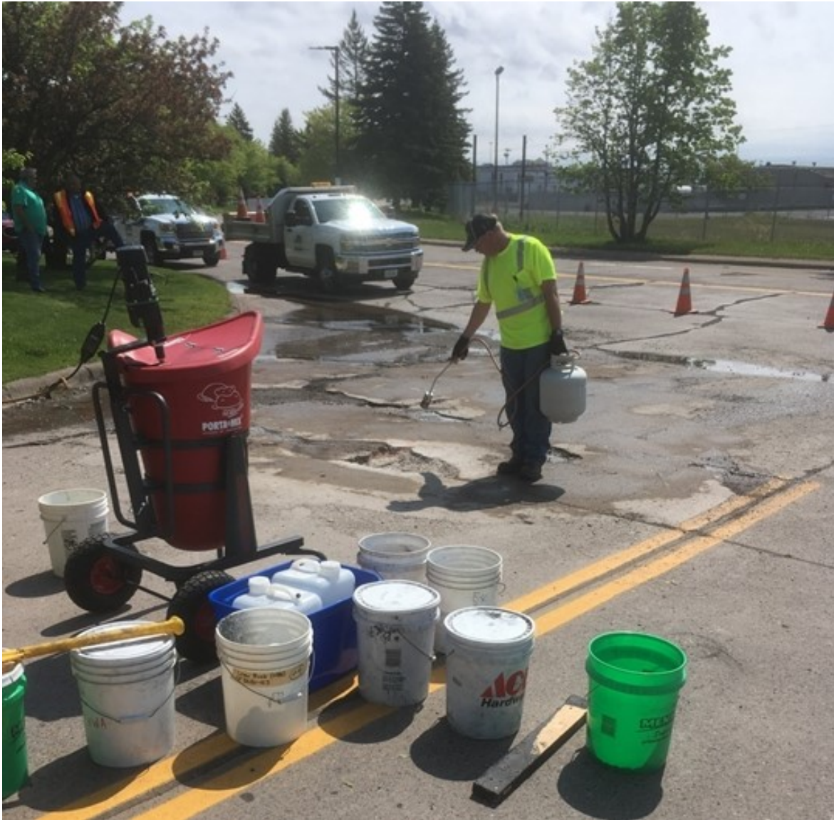
Figure 2.41 Pothole repair setup and preparation, June 6, 2018, Duluth field trial location.
