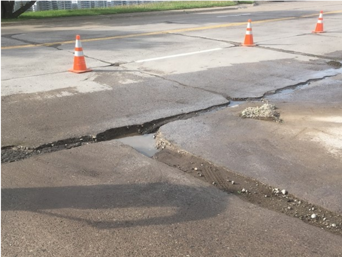
Figure 2.43 Target pavement repair: June 7, 2018, Duluth field trial location.
