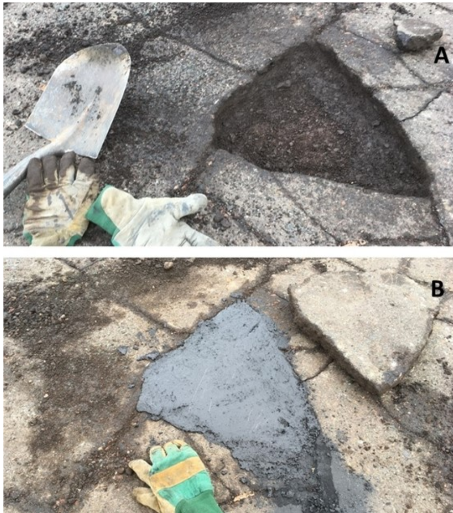
Figure 2.63 November 20, 2017, cold temperature pothole test at NRRI; before (A) and after (B).
