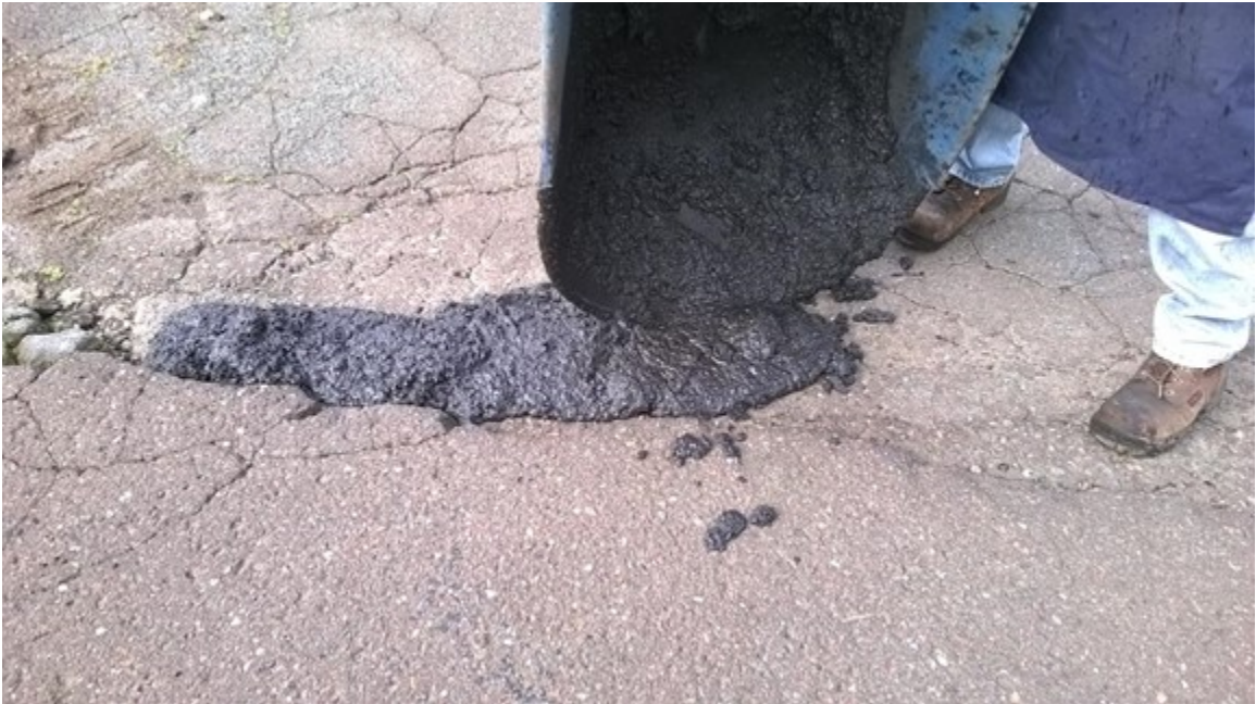
Figure 2.26 Pouring October 5, 2017, test repair in NRRI parking lot.
