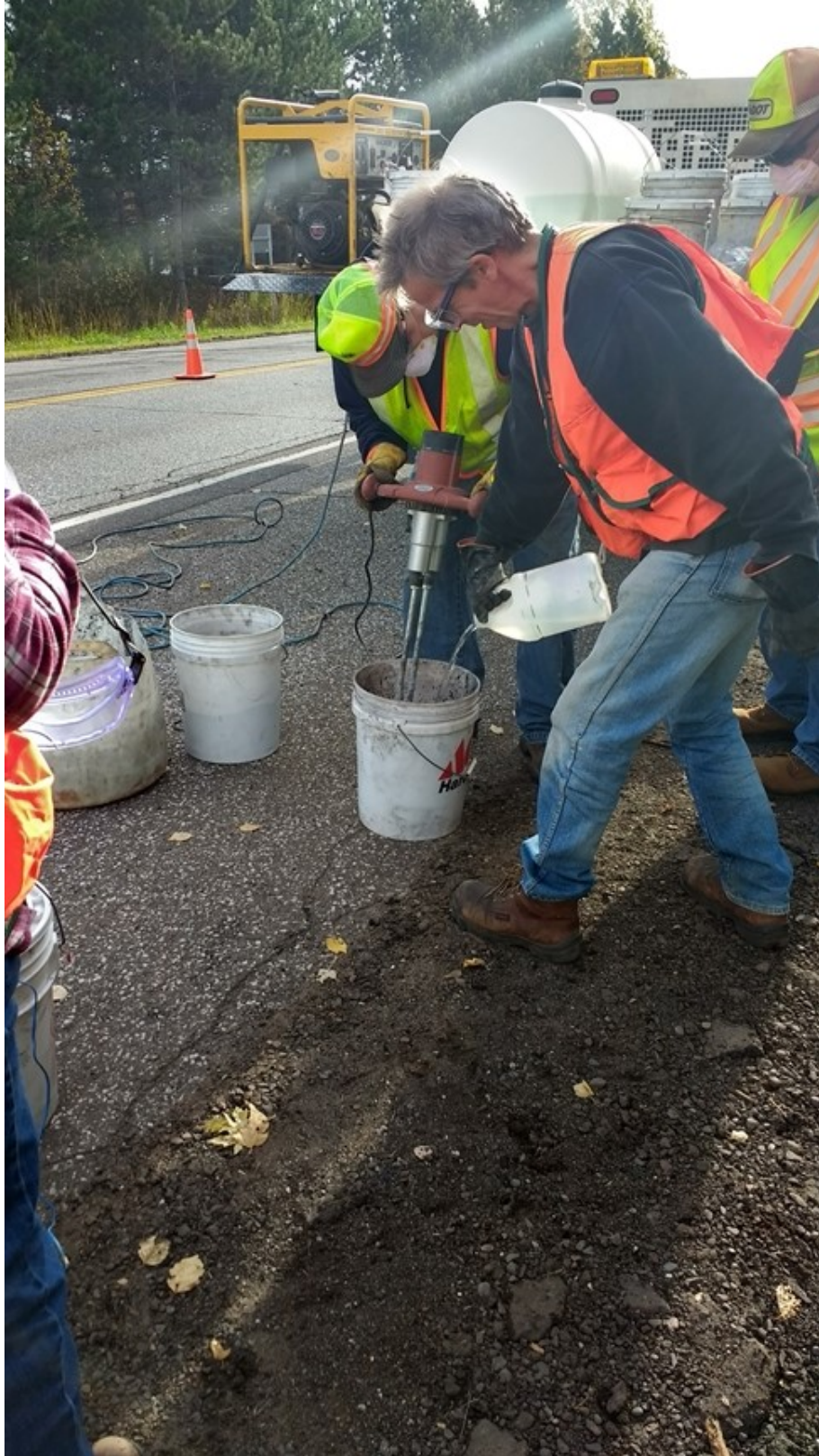
Figure 2.31 Preparing repair material with MnDOT crew, October 18, 2017.
