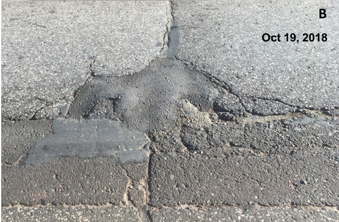
Figure 2.73 Condition of June 20, 2018 Proctor repairs on June 20, 2018 (A) and October 19, 2018 (B).
