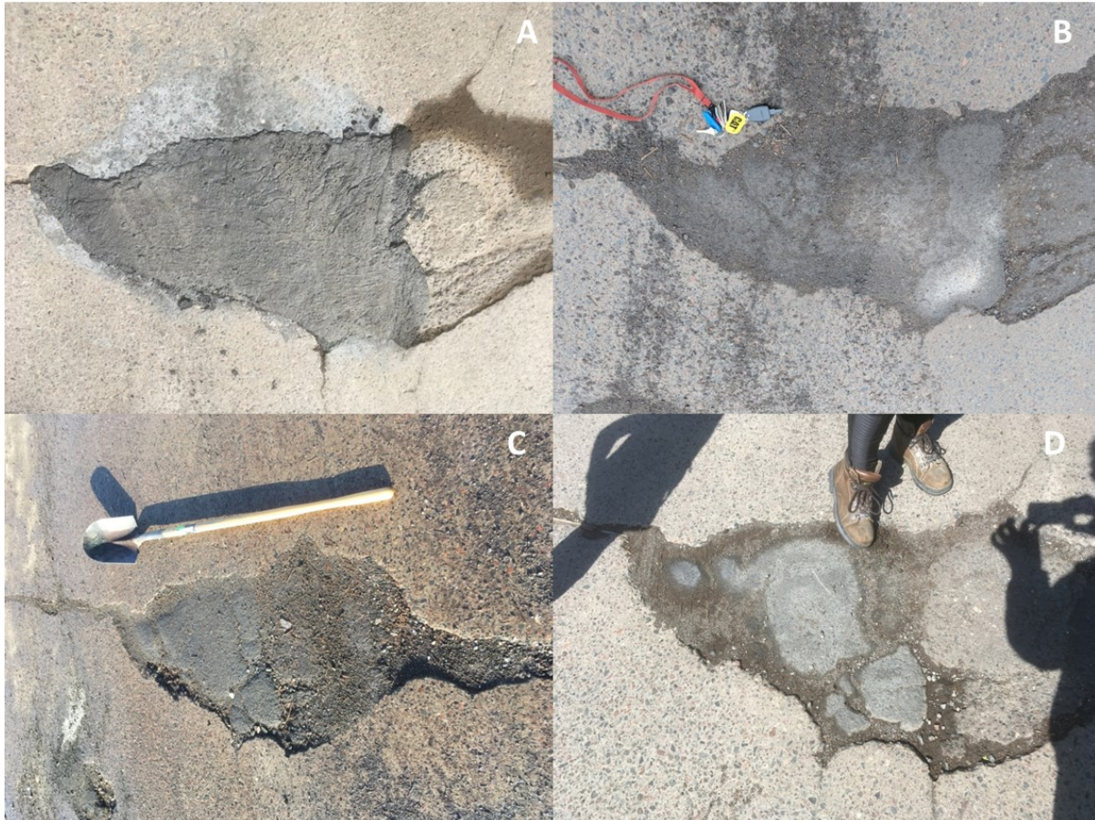
Figure 2.78 Condition of June 6, 2018, city of Duluth field trial repair on: (A) June 7, 2018; (B) December 12, 2018; (C) March 19, 2019; and (D) August 29, 2019.
