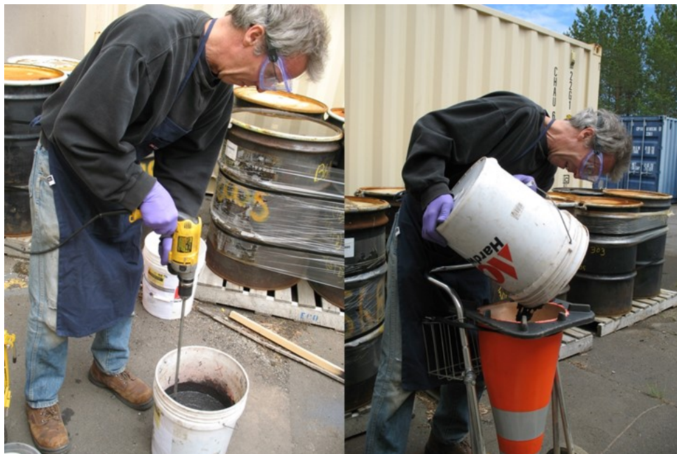
Figure 2.8 Repair compound mixing and pouring for May 24, 2017, test.
