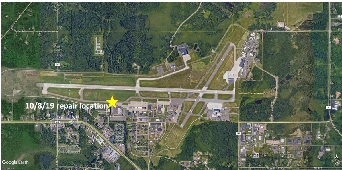
Figure 2.95 Location of October 8, 2019, Duluth Airport Authority taxiway repair (Image source: Google Earth).
