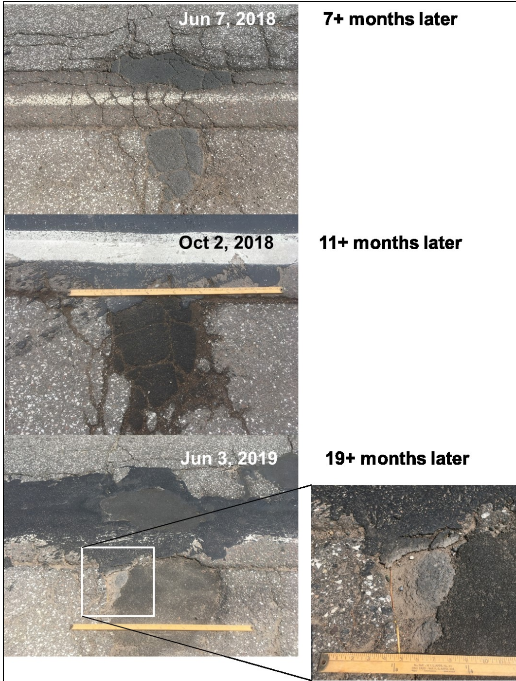
Figure 2.72 Condition of the October 18, 2017 Proctor/Hwy 2 repair: from June 7, 2018 to June 3, 2019.
