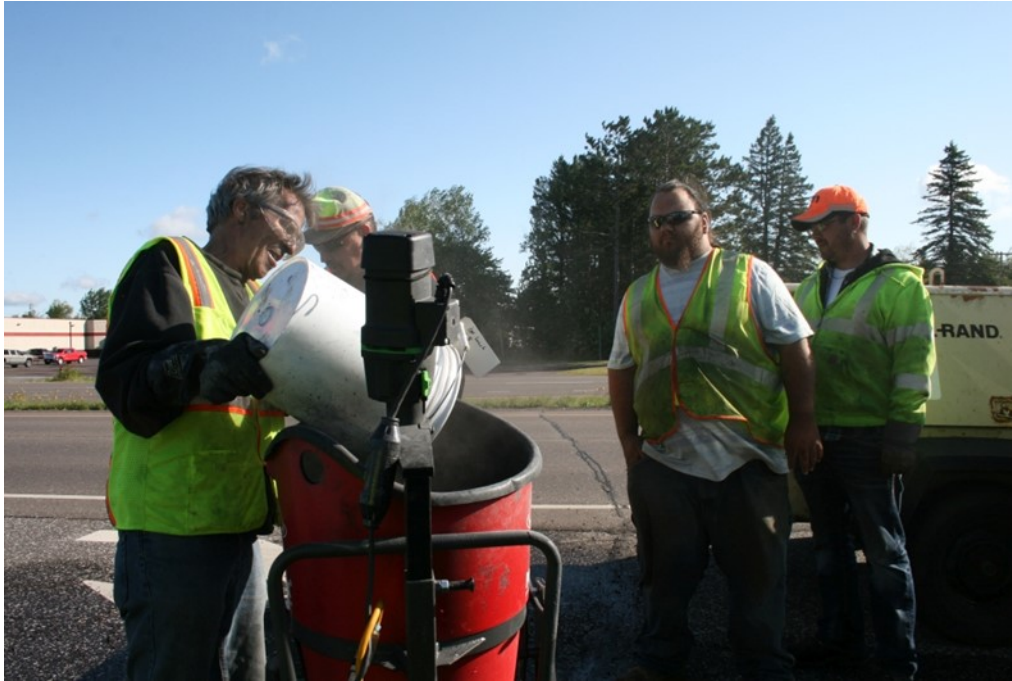
Figure 2.85 Adding and mixing repair compound components at the U.S. Highway 53 field trial location.
