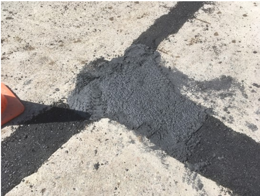
Figure 2.46 Completed repair: June 7, 2018, Duluth field trial location.
