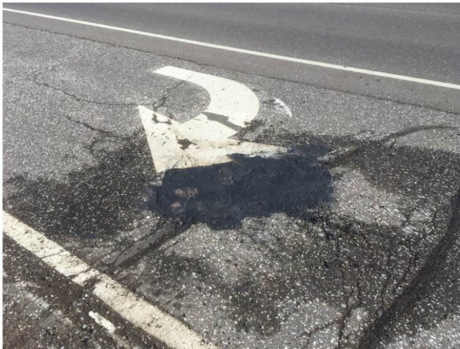
Figure 2.89 Completed repair at the U.S. Highway 53 field trial location (August 29, 2019).
