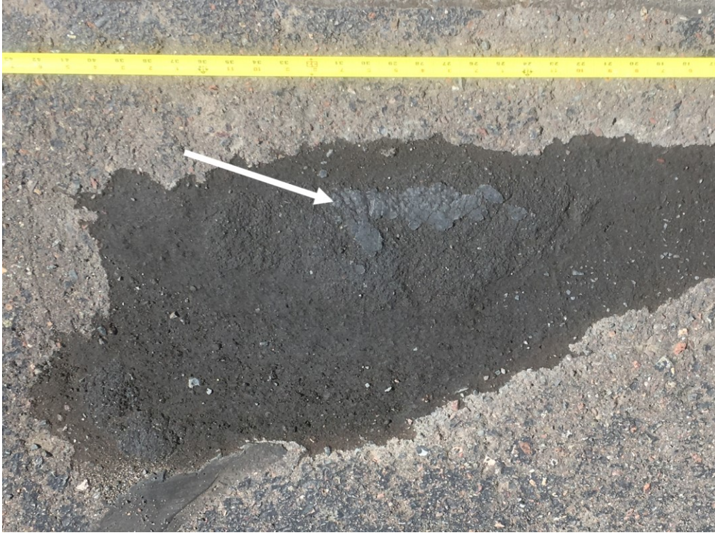
Figure 2.66 Close-up of April 22, 2018 repair, with arrow pointing to original remaining surface.
