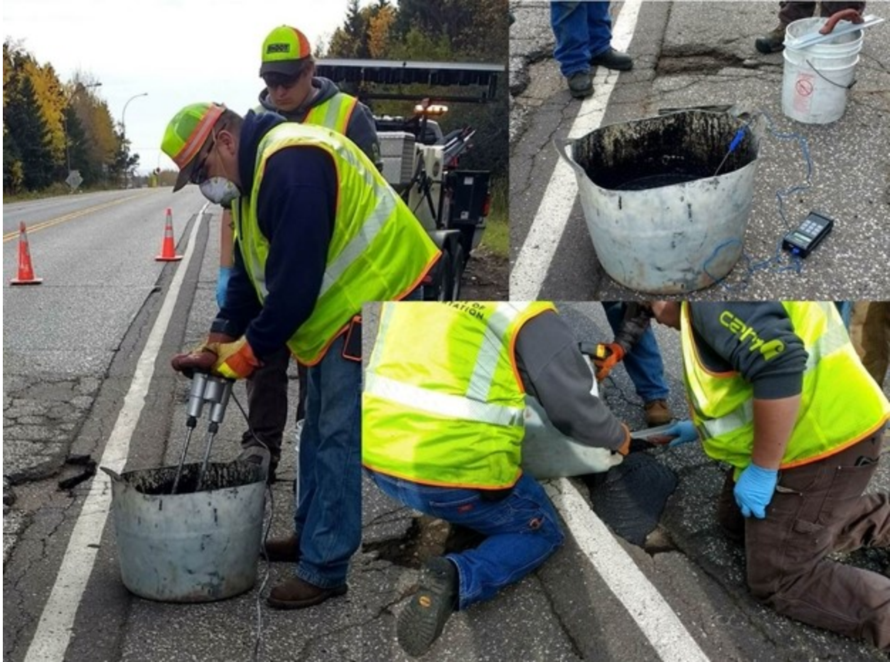
Figure 2.32 MnDOT crew preparing and installing repair compound, October 18, 2017.
