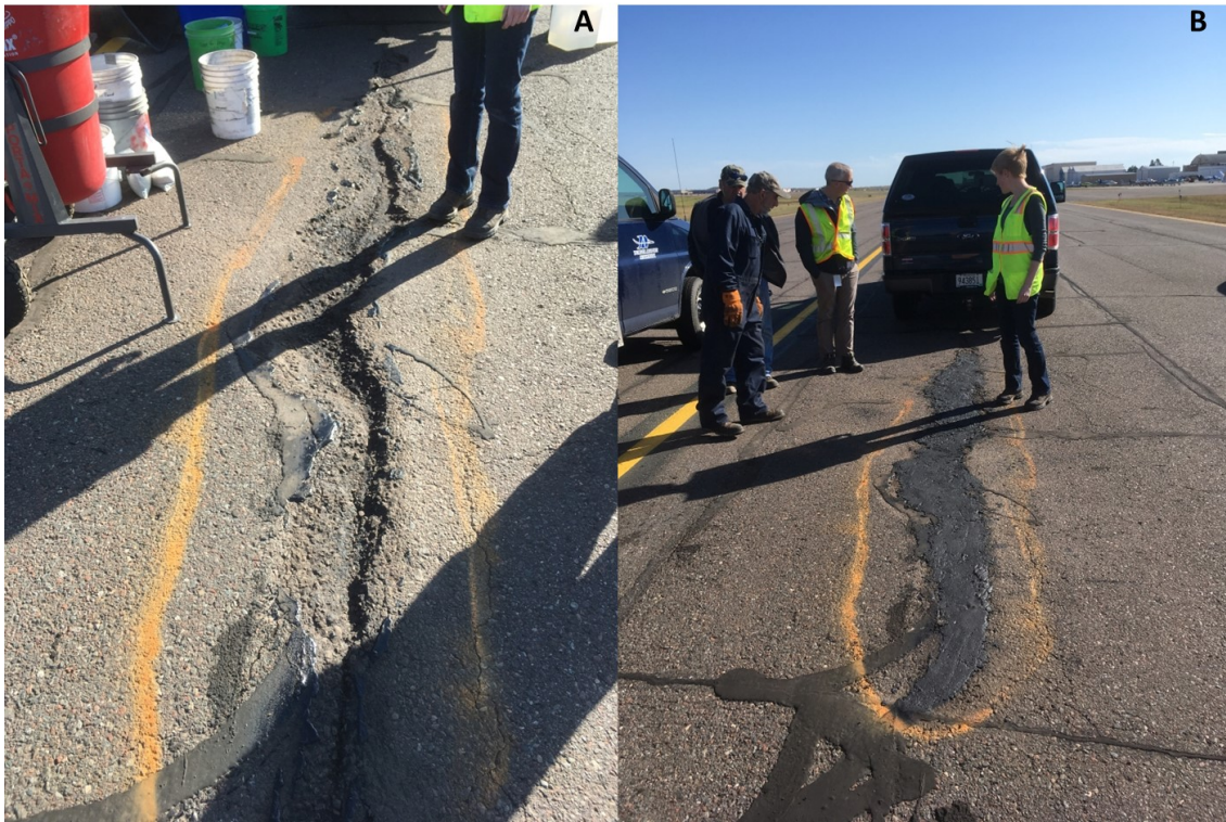
Figure 2.98 Duluth Airport Authority taxiway repair before (A) and after (B); October 8, 2019.
