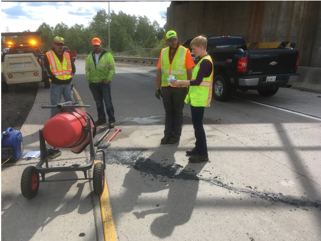
Figure 2.93 Completed repair at U.S. Highway 2 and I-35 Thompson Hill field trial location, showing blue portable generator and “Mega Hippo” mixer on the left, and MnDOT District 1 crew with the NRRRI’s Sara Post.
