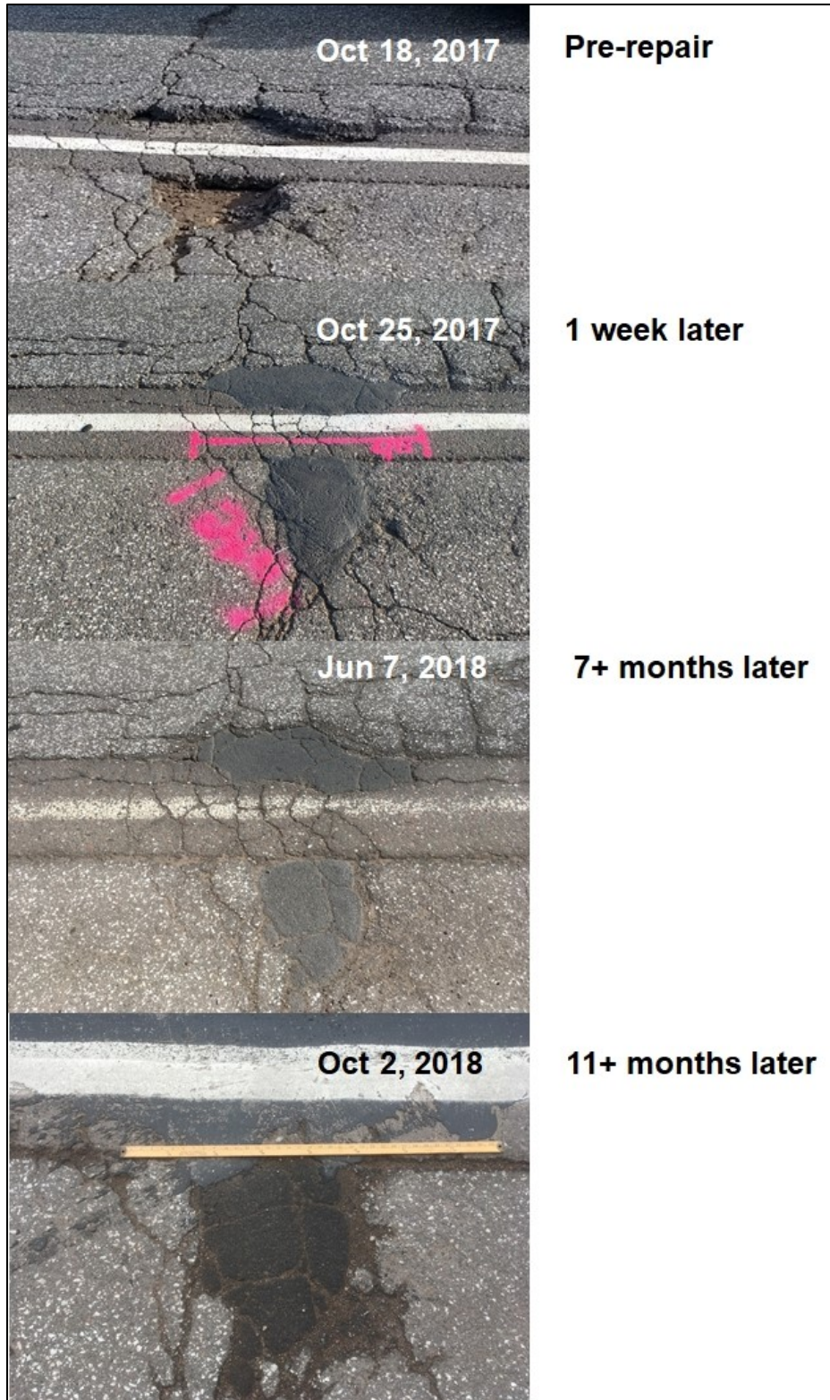
Figure 2.71 Condition of Proctor/Hwy 2 repair from October 18, 2017, to October 2, 2018.
