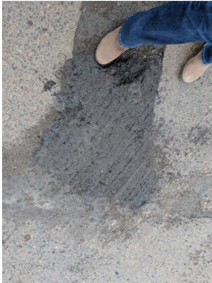
Figure 2.76 Condition of June 7, 2018, Duluth field trial repair on December 12, 2018, showing deterioration.
