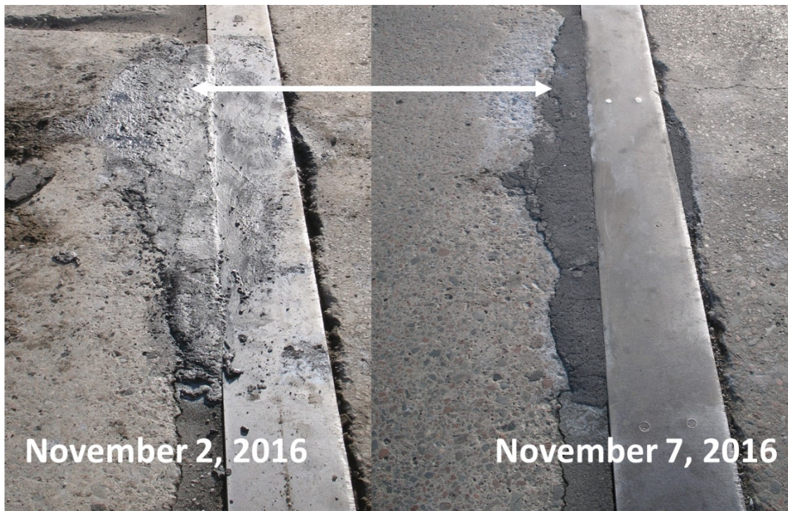
Figure 2.16 Condition of repair made at Mesaba Avenue expansion joint: November 2 (left); and November 7 (right), 2016.
