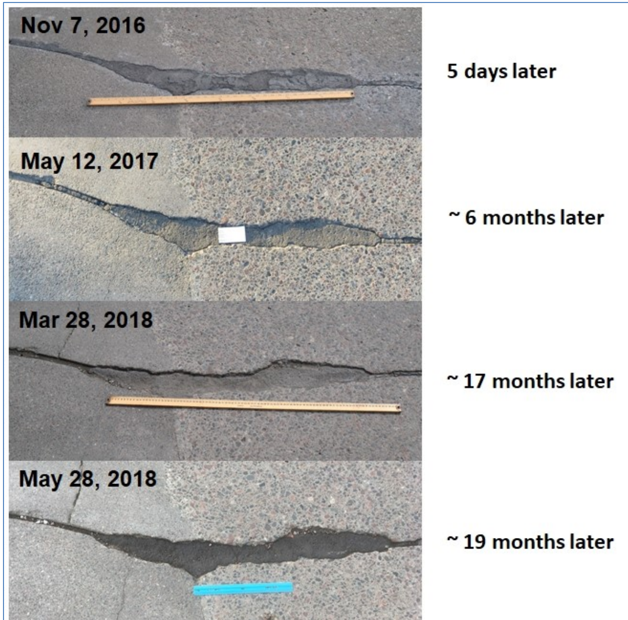
Figure 2.59 Condition of Mesabi Avenue crack repair from November 7, 2016, to May 28, 2018.
