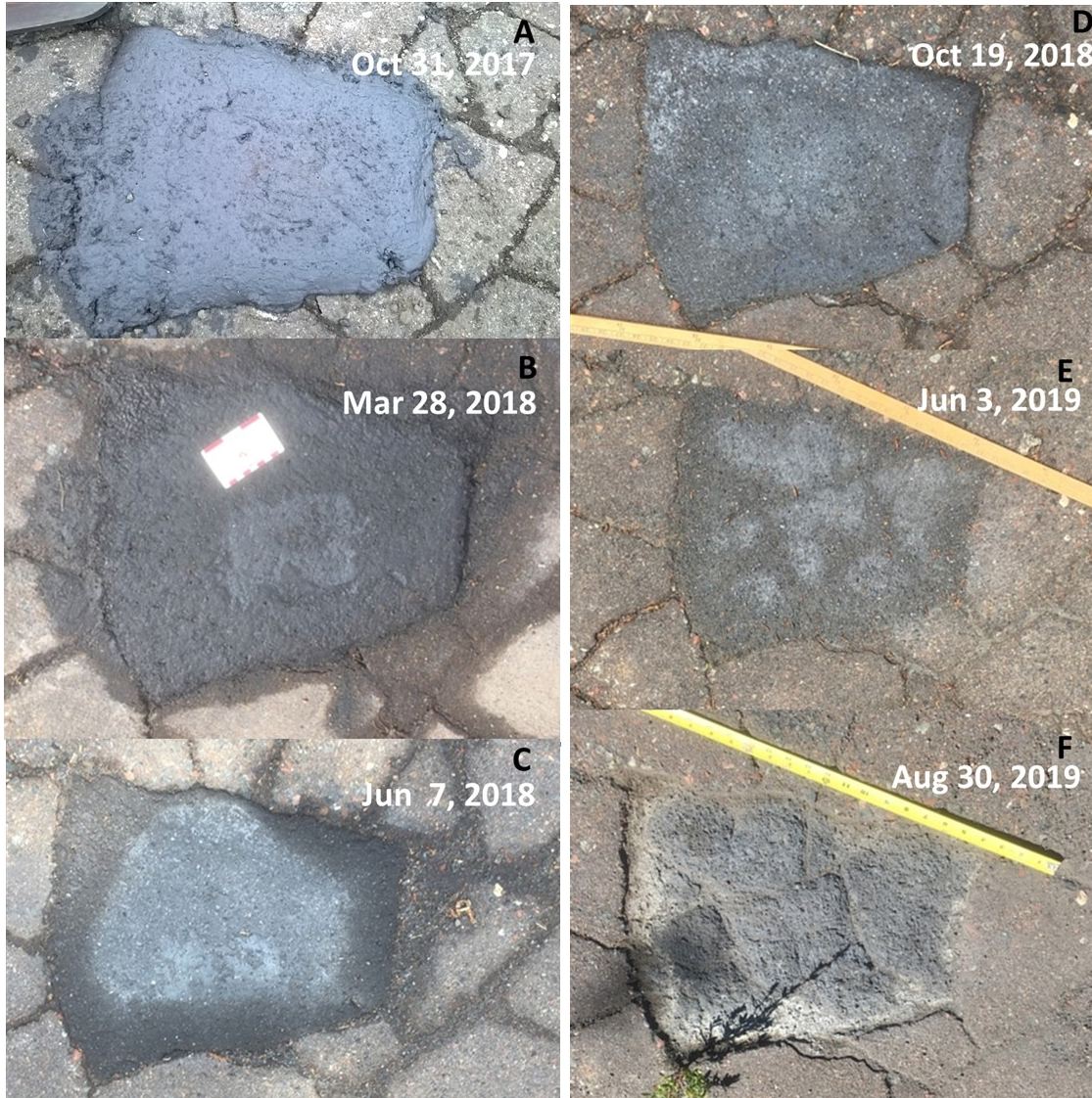
Figure 2.62 October 31, 2017, NRRI parking lot repair: Completed repair (A); and conditions of repair on March 28, 2018 (B); June 7, 2018 (C); October 19, 2018 (D); June 3, 2019 (E); and August 30, 2019 (F).
