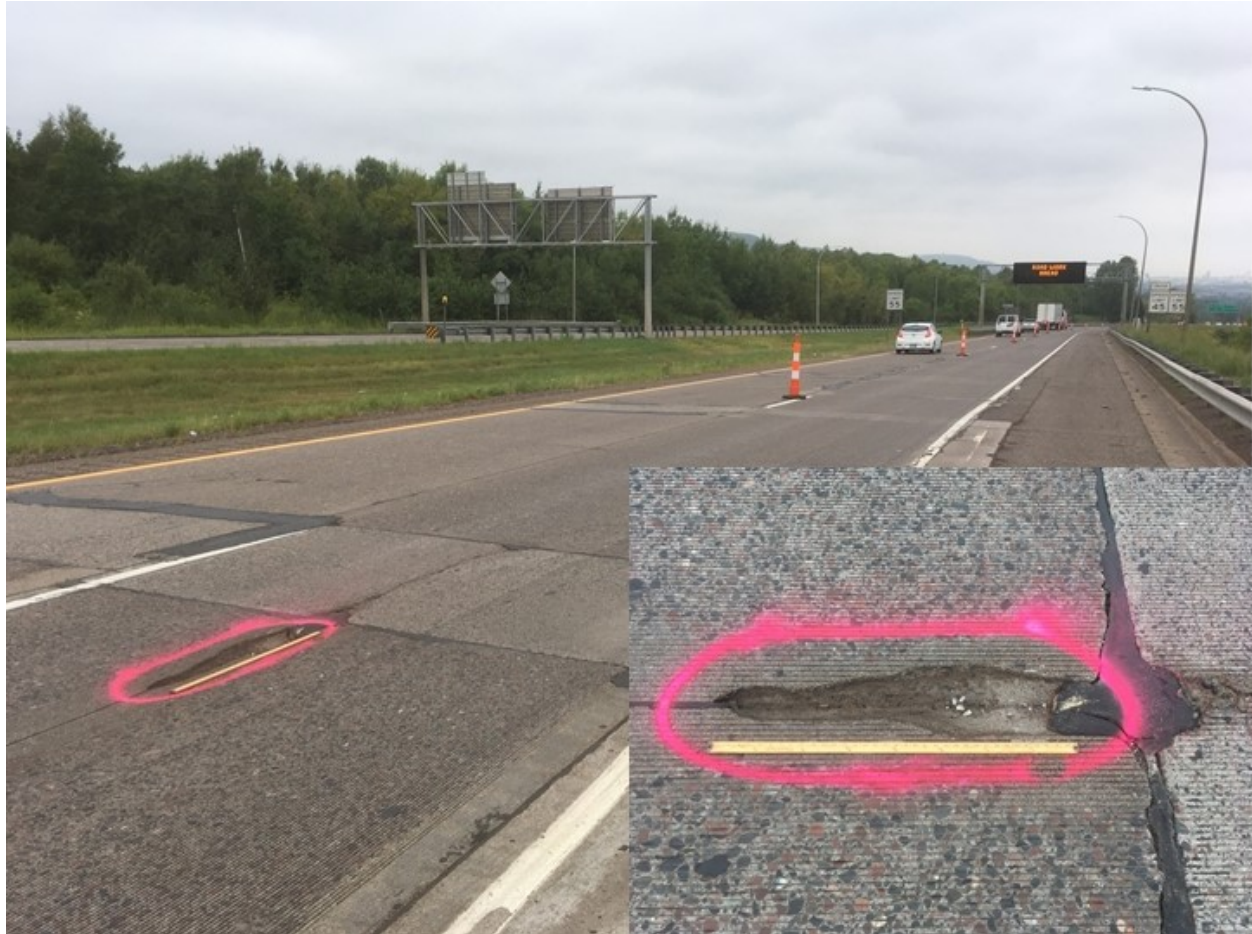
Figure 2.52 Potential southbound I-35 repair: Thompson Hill, Duluth (inset shows detail).
