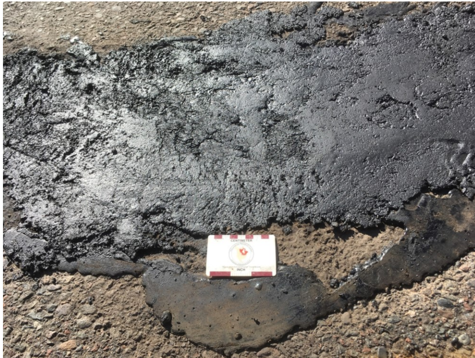
Figure 2.99 Closeup of finished taxiway repair and adjacent mastic.
