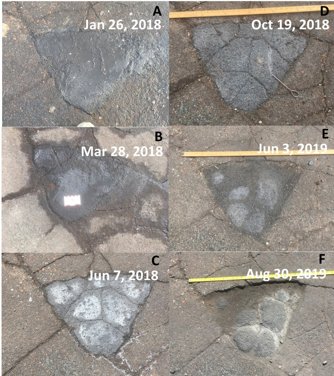
Figure 2.64 Condition of the November 20, 2017 repair from January 26, 2018 to August 30, 2019.
