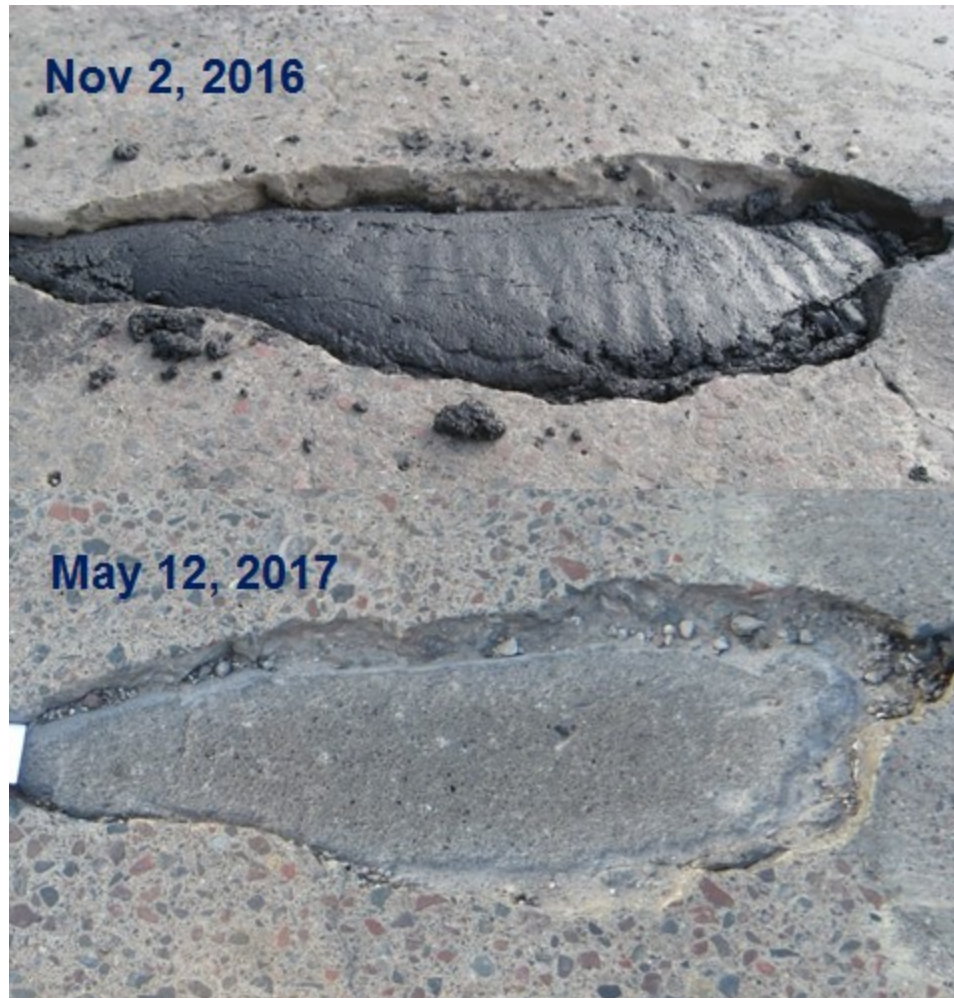
Figure 2.17 Condition of Mesaba Avenue repair following installing on November 2, 2016 (top photo) and on May 12, 2017 (bottom photo).
