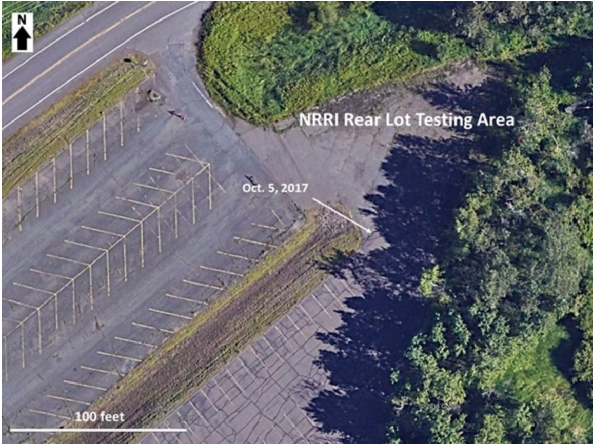
Figure 2.25 More detailed image of NRRI rear parking lot test area, with arrow pointing to October 5, 2017, repair location. (Image source: Google Earth)
