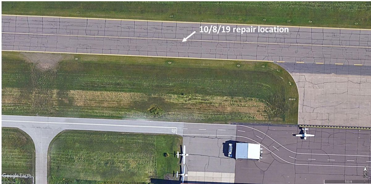
Figure 2.96 Closer view of October 8, 2019, Duluth Airport Authority taxiway repair location (Image source: Google Earth).
