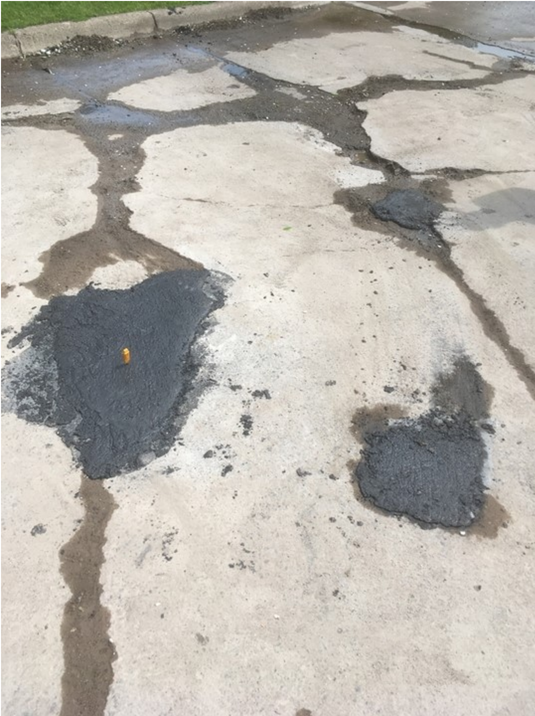
Figure 2.42 Finished Batch 2 repairs: June 6, 2018, Duluth field trial location.
