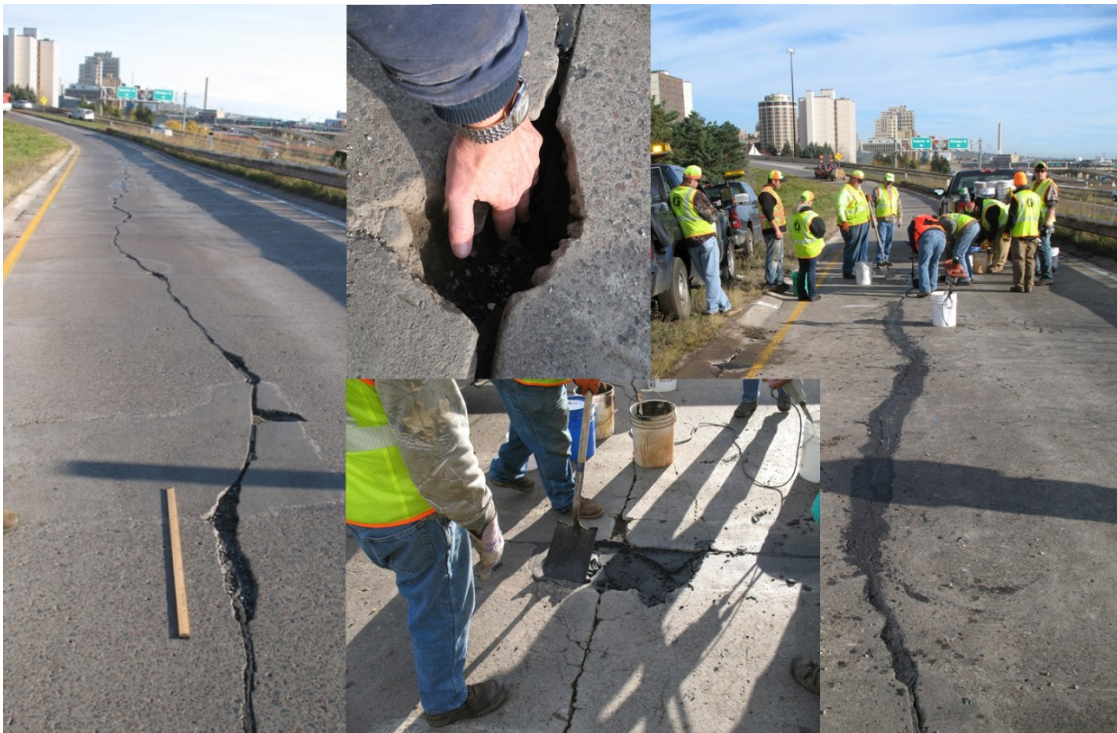
Figure 2.15 Pavement condition and initial repairs: Mesaba Avenue, Duluth - November 2, 2016
