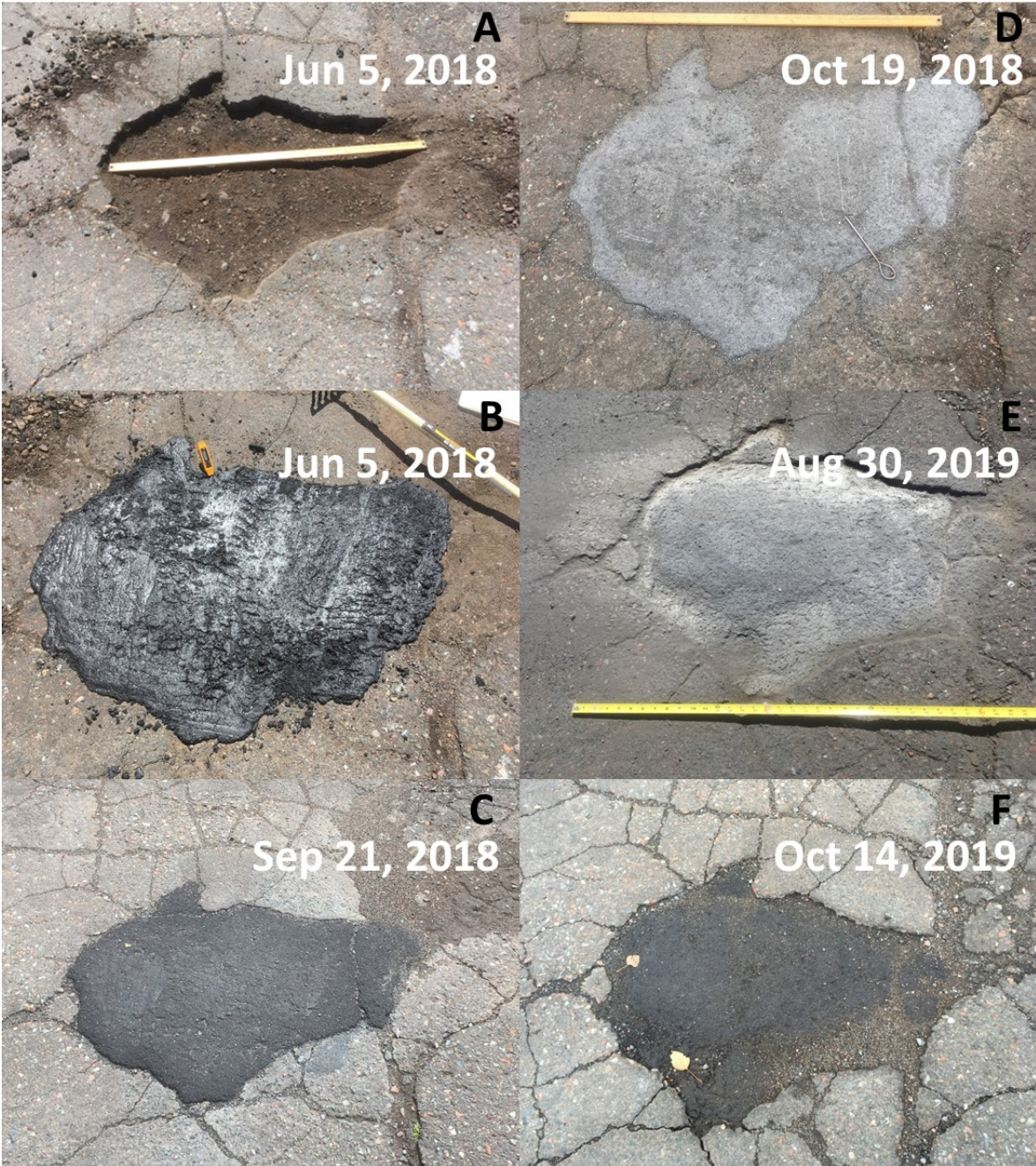
Figure 2.68 Condition of the June 5, 2018 repair from June 5, 2018 (A and B) to October 14, 2019 (F).
