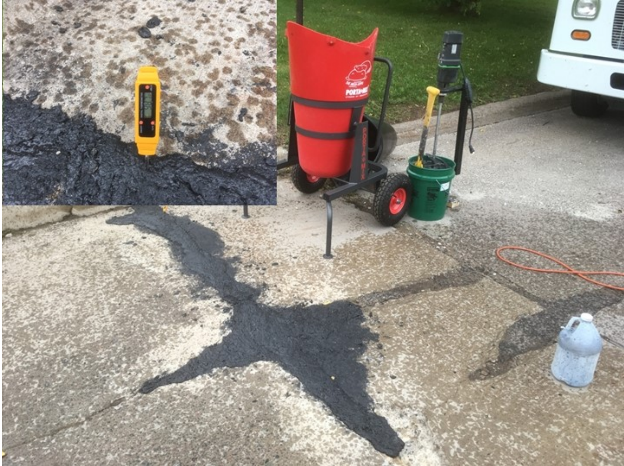
Figure 2.48 Completed repair: September 27, 2018, Duluth field trial location (inset showing curing temperature).
