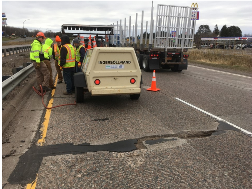
Figure 2.103 MnDOT District 1 crew and equipment at Repair #1 location, southbound I-35 and Boundary Avenue test location (Hole 1 in foreground): October 31, 2019.
