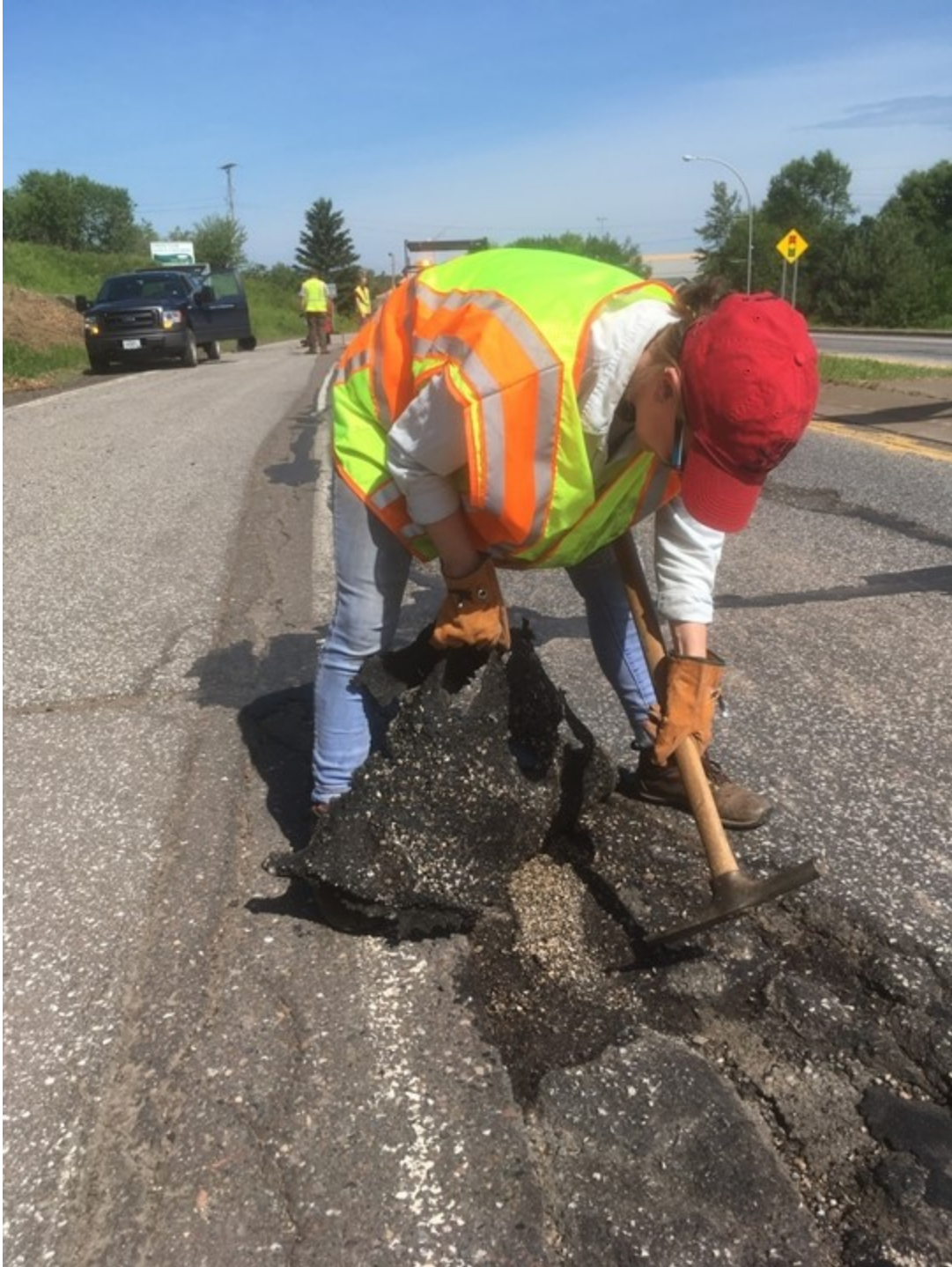
Figure 2.50 Delaminating mastic repairs, Proctor, MN, field trial site: June 20, 2018.
