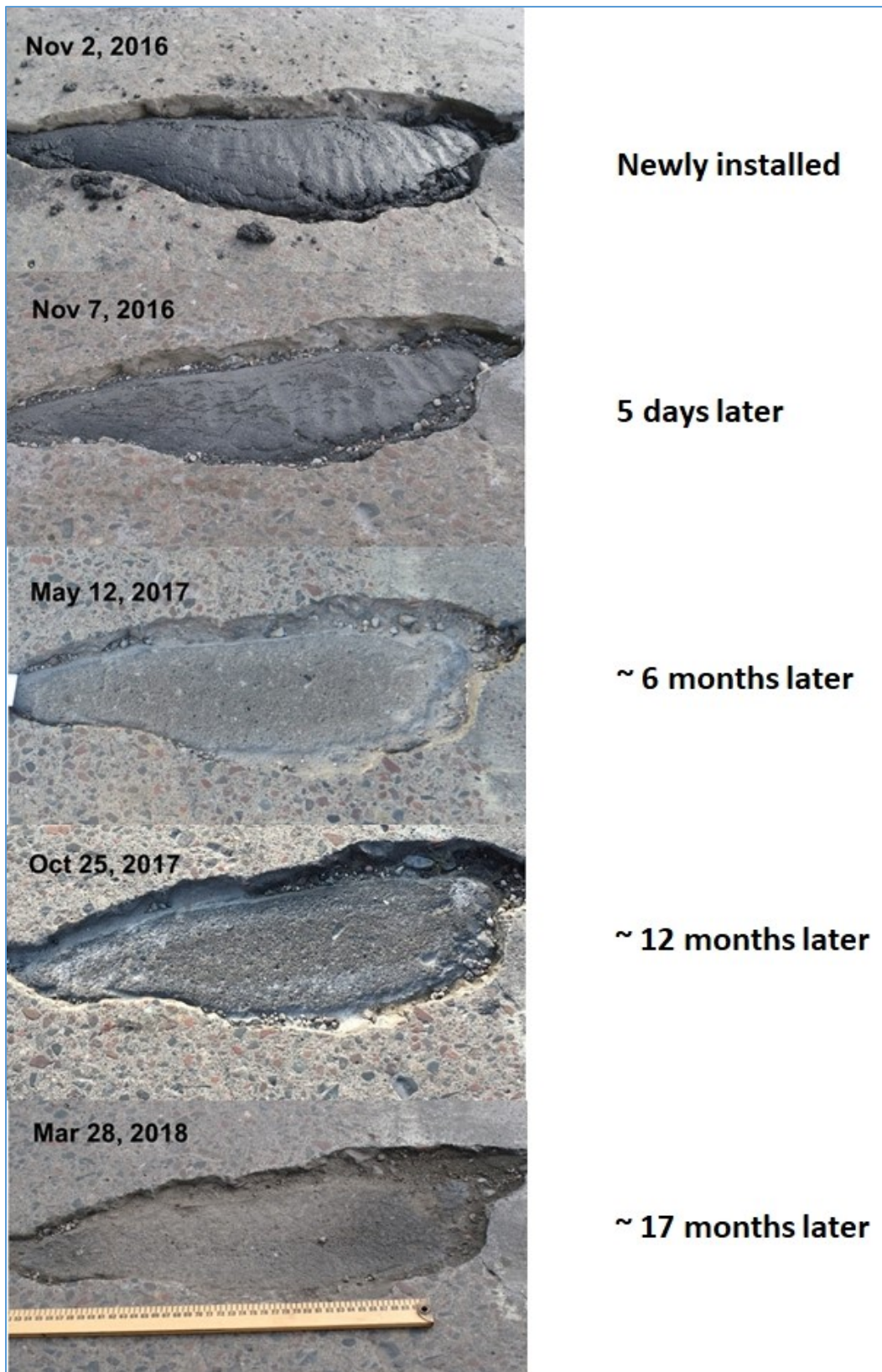
Figure 2.58 Condition of Mesaba Avenue repair from November 2, 2016, to March 28, 2018.
