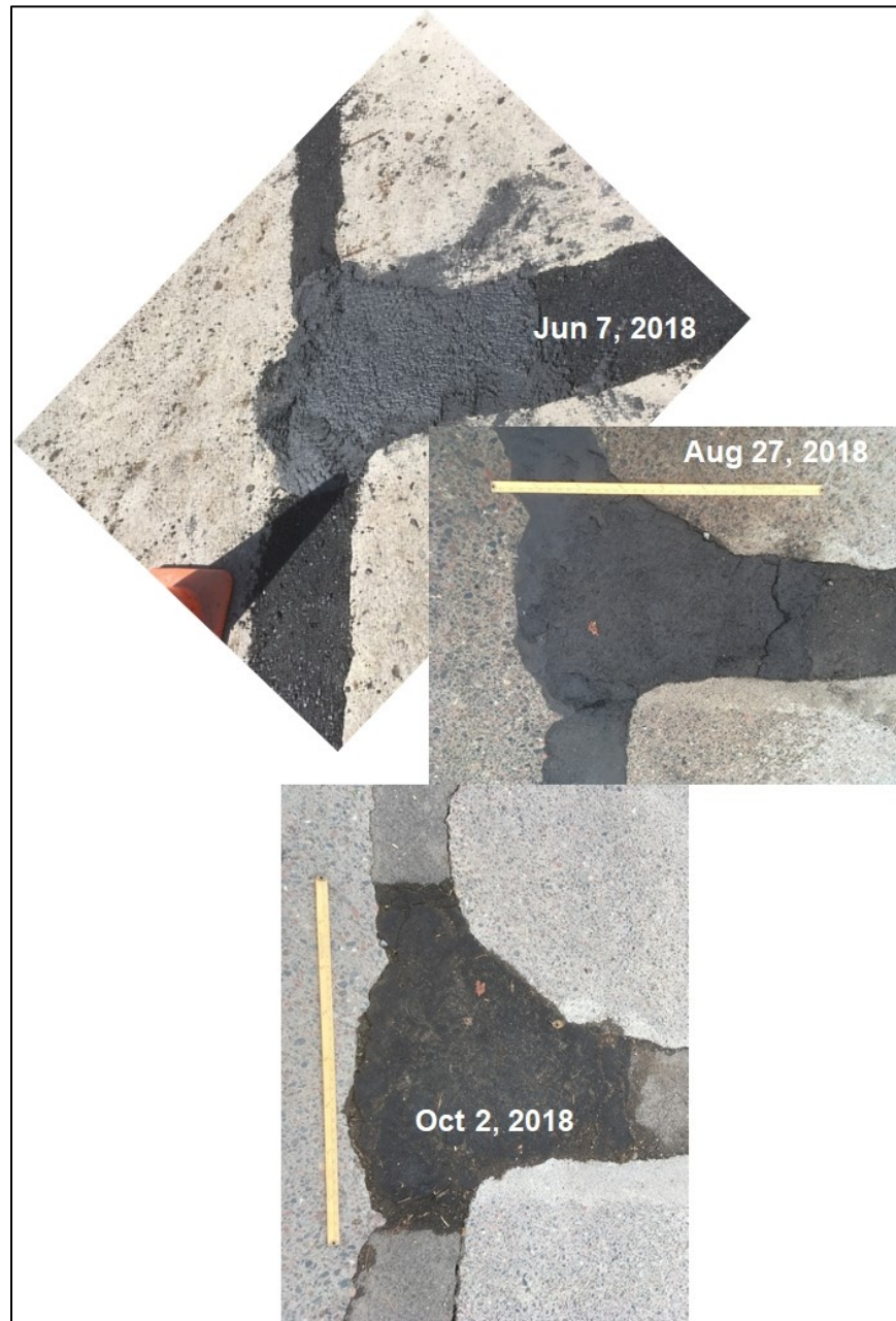
Figure 2.74 Condition of June 7, 2018, city of Duluth field trial repair through October 2, 2018.
