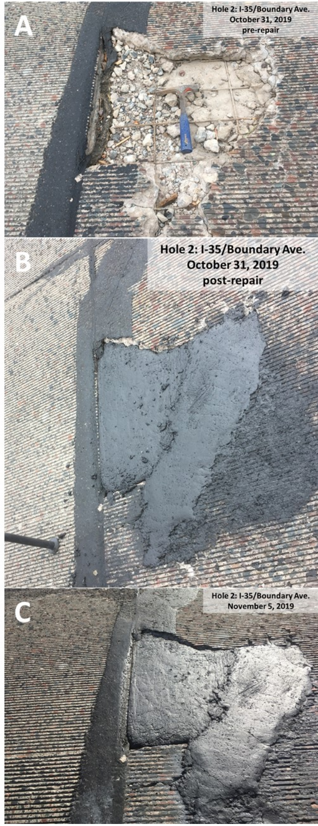
Figure 2.105 Hole 2 repair at I-35/Boundary Avenue location: pre-repair (A) and post-repair (B) on October 31, 2019; and on November 5, 2019 (C).
