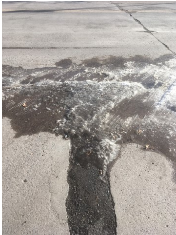
Figure 2.75 Ice-covered condition of June 7, 2018, Duluth field trial repair on November 17, 2018.
