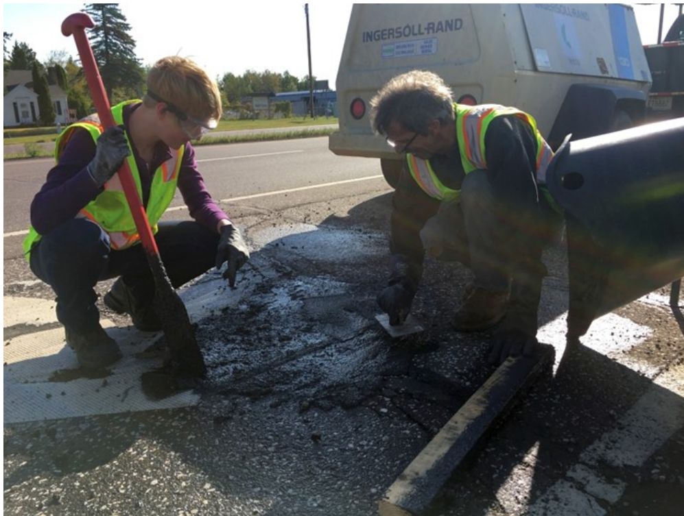
Figure 2.87 Finishing the completed repair at the U.S. Highway 53 field trial location.
