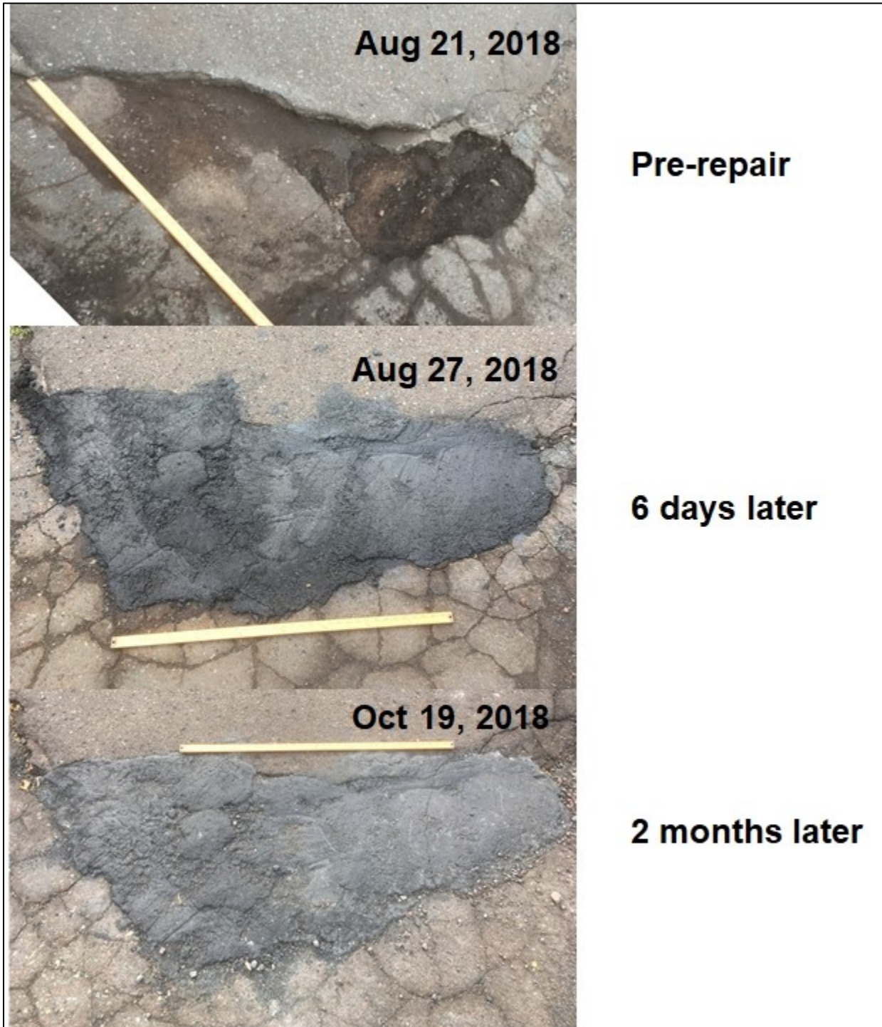
Figure 2.69 August 21, 2018, NRRI parking lot test repair condition through October 19, 2018 (yard stick for scale).
