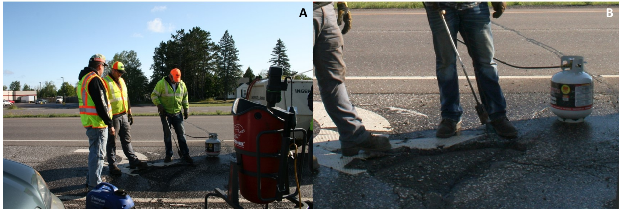
Figure 2.84 MnDOT District 1 crew preparing pothole for repair (A) and driving moisture from the pothole with a propane torch (B).
