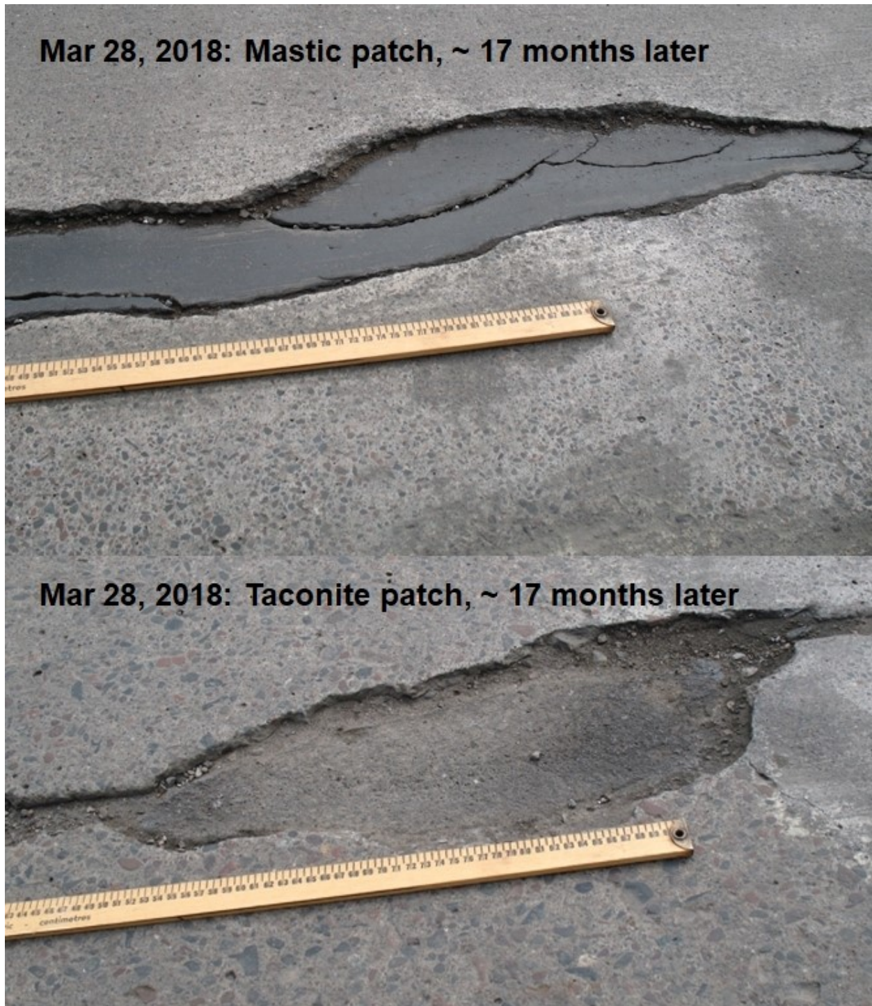
Figure 2.60 Comparison of mastic and taconite patch repairs after 17 months (as of March 28, 2018).
