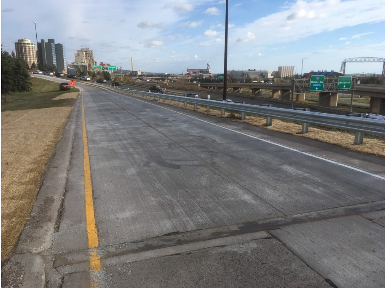
Figure 2.61 Rehabilitated Mesaba Avenue pavement as of October 19, 2018.
