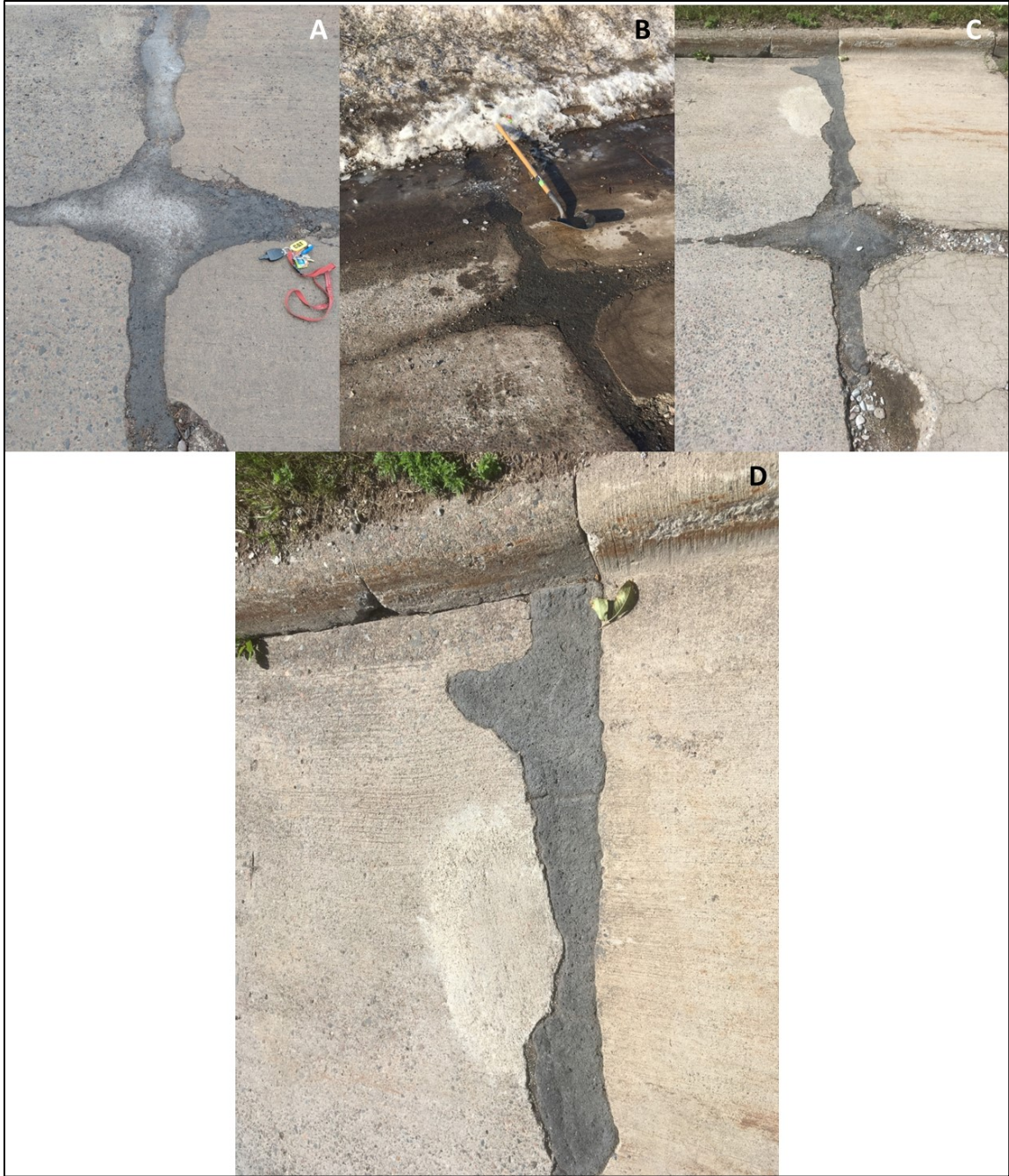
Figure 2.79 Condition of September 27, 2018, city of Duluth field trial repair on: (A) December 12, 2018; (B) March 19, 2019; (C) August 29, 2019; and (D) August 29, 2019 (close-up).
