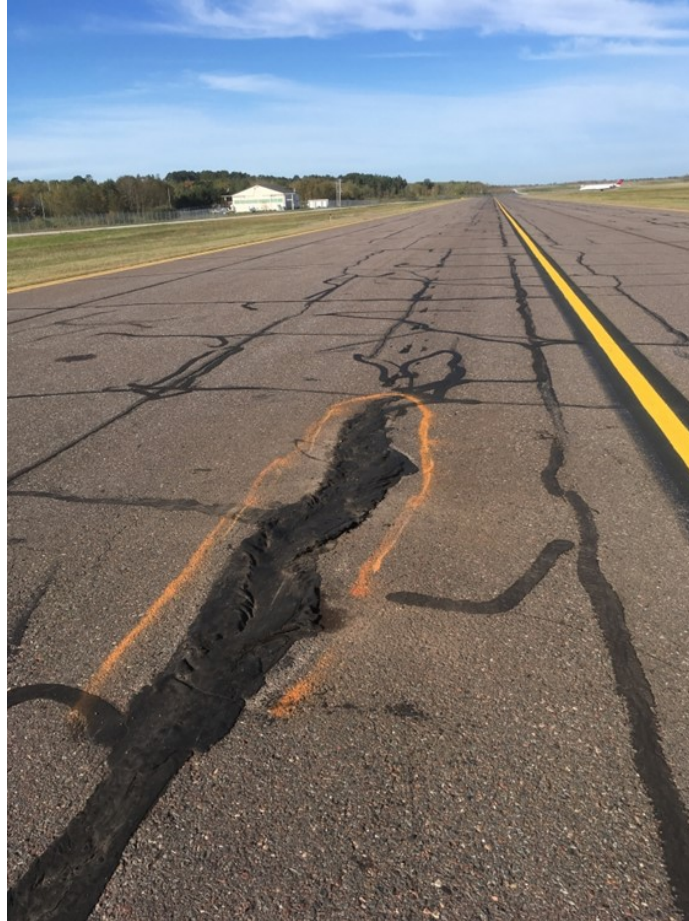
Figure 2.97 Target pavement distress and condition of mastic repair on airport taxiway (September 27, 2019).
