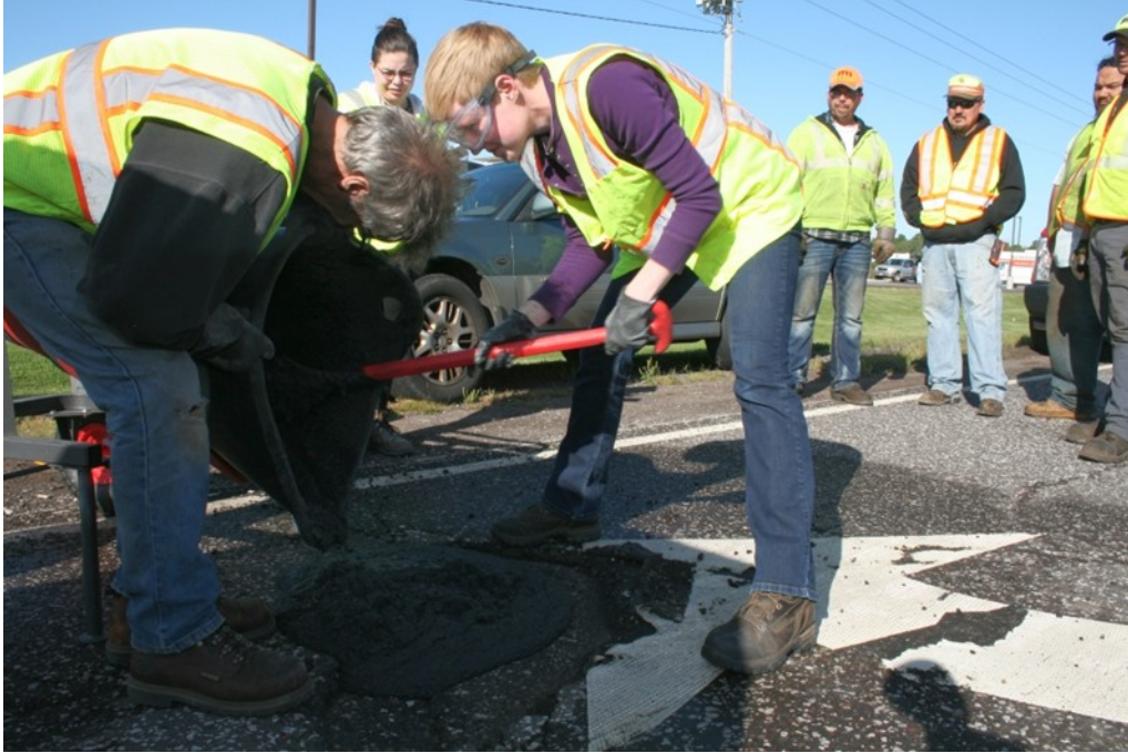
Figure 2.86 Dispensing the repair compound into the pothole at the U.S. Highway 53 field trial location.
