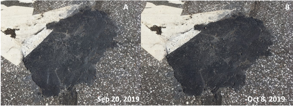
Figure 2.90 Follow-up photographs of the August 29, 2019, U.S. Highway 53 field trial repair on September 20, 2019 (A) and October 8, 2019 (B).
