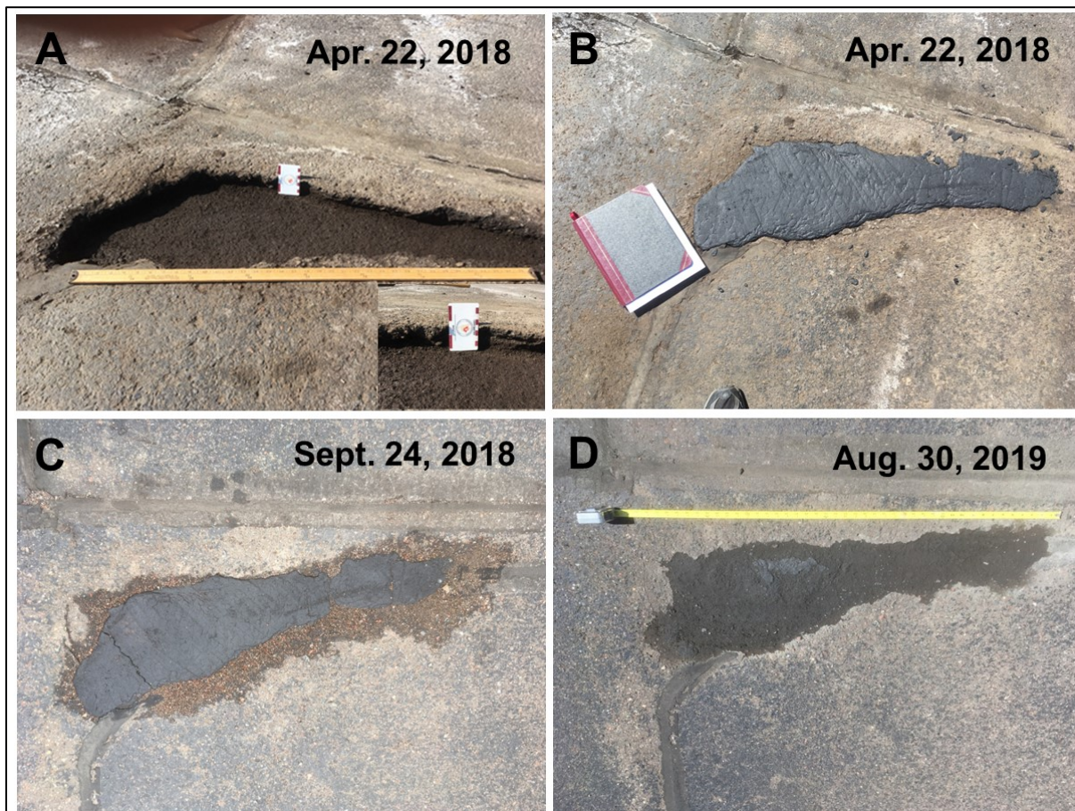
Figure 2.65 April 22, 2018 NRRI parking lot repair: A) prepared hole, with inset photo showing depth; B) completed repair; C) condition of repair on September 24, 2018; and D) condition of repair on August 30, 2019.
