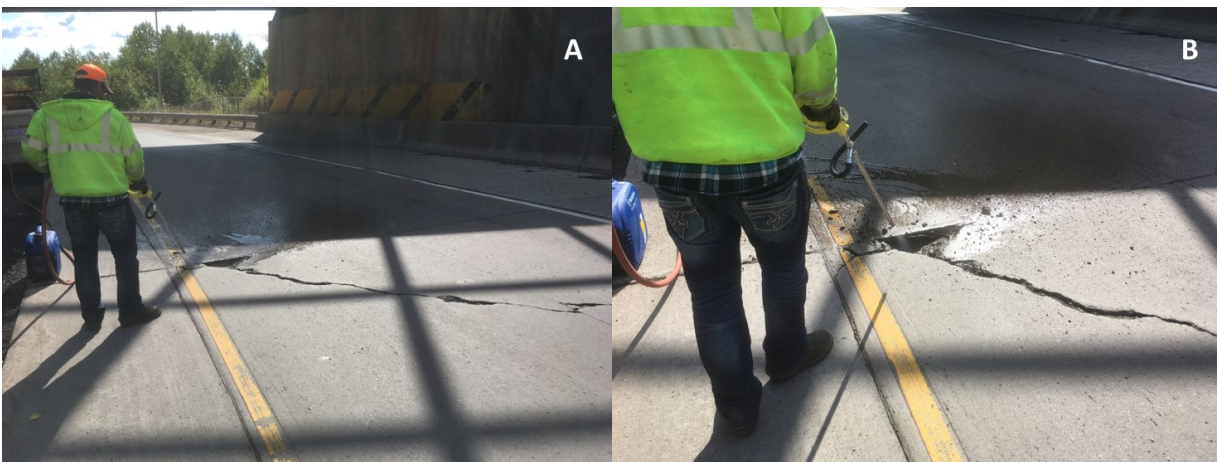
Figure 2.92 MnDOT District 1 personnel removing loose debris from pothole with compressed air at U.S. Highway 2 and I-35 Thompson Hill field trial location (A); closer view (B) on August 29, 2019.
