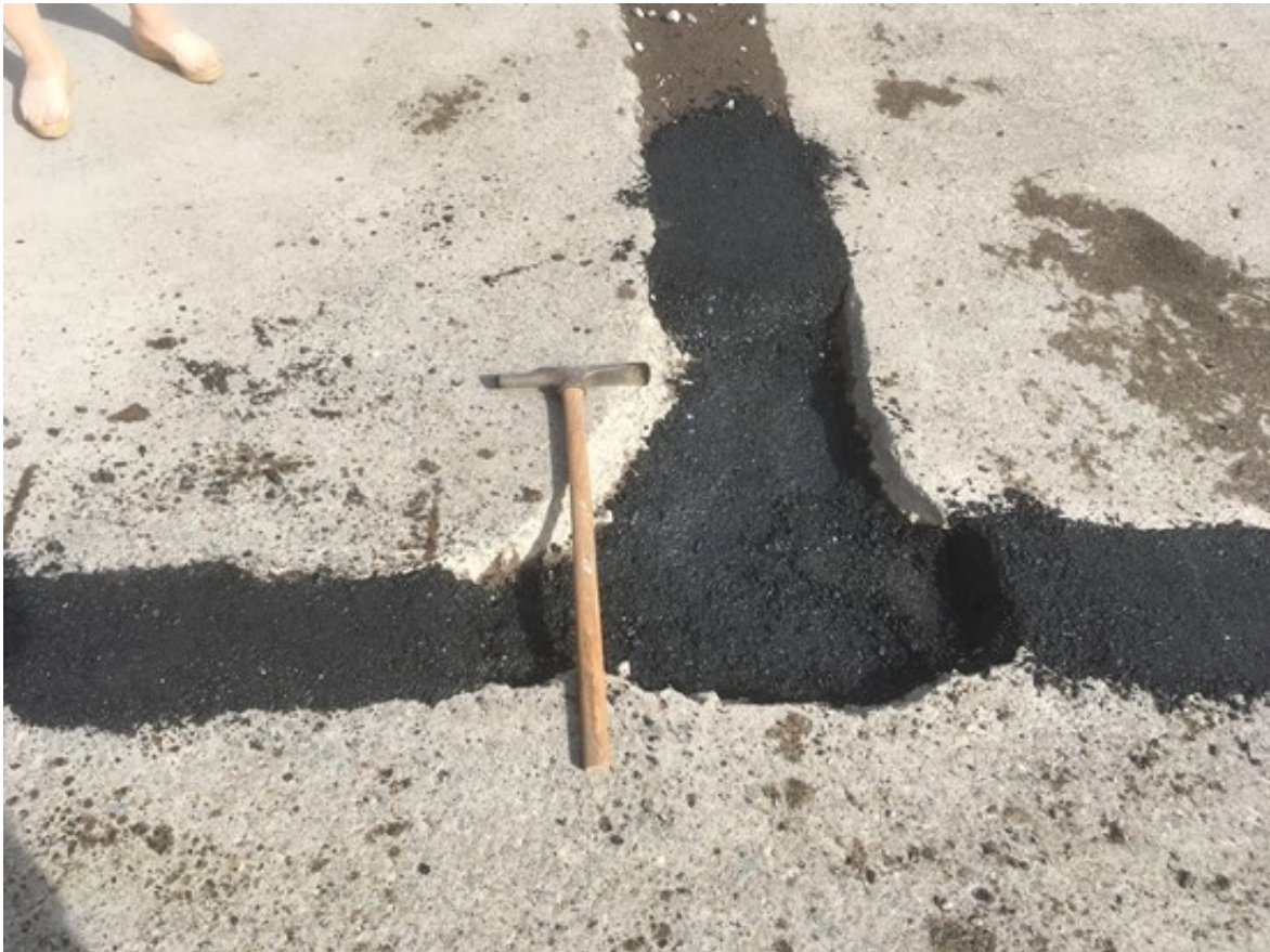
Figure 2.45 Target pavement repair prepared with hot mix asphalt: June 7, 2018, Duluth field trial location.
