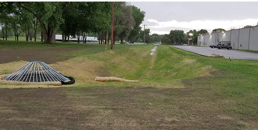
Mitigation measures include a flood control ditch.
