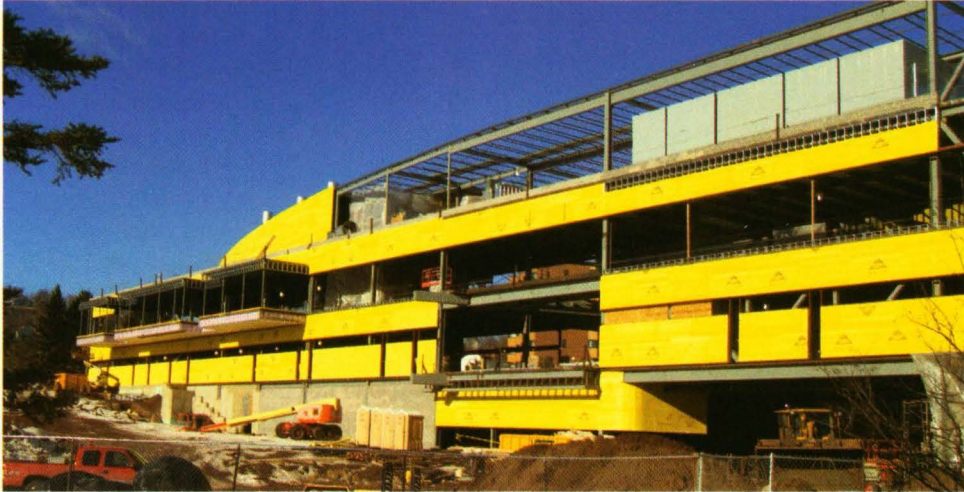
Above: The Swenson Science Building construction began in early 2003. The expected completion is 2005.
