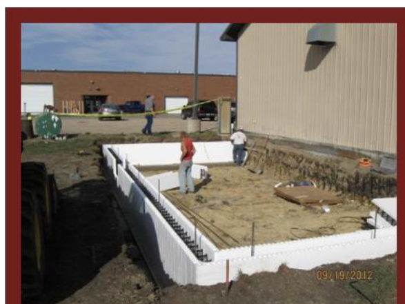
The process of constructing the foundation
