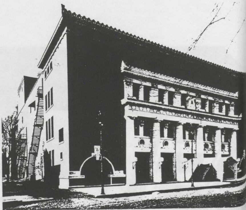
First Minneapolis Auditorium, about 1905
