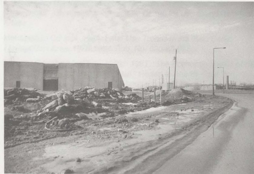
Industrial and commercial infill have replaced former rail land along Energy Park Drive in St. Paul.
