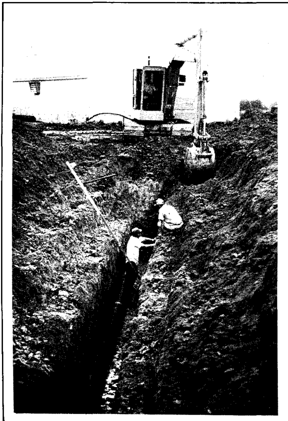
Figure 6. Chain-trencher excavating and installing 12-in. diameter tubing for a 1,600-cfm capacity system in Menard County, Illinois. Three to 4 ft. of soil was removed, using a bulldozer before the trencher was used to install the tubing an additional 6 ft. into the soil.
