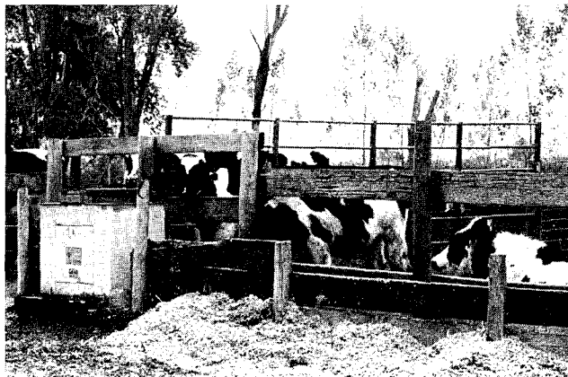
Grounding conductors for electrically heated waterers must be securely bonded to provide a low resistance path to ground.
