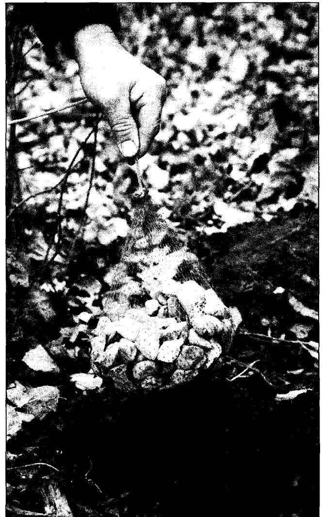
Figure 5. If the gravel which protects the hole bottom from scouring is contained in a nylon mesh bag, it can be removed and reused.
