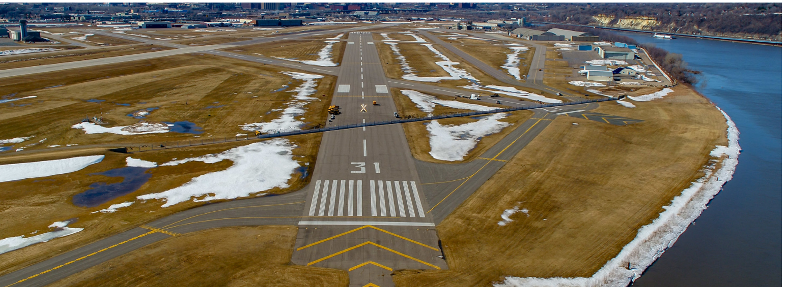
The deployable floodwall during installation in March 2019 at the St. Paul Downtown Airport. (Photo courtesy of the Metropolitan Airports Commission.)
