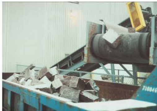
Figure 28. Cold Spring Granite cut-off blocks transported via conveyor to demolition container.
