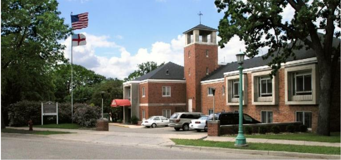
Figure 11. Exterior of Building B. Source from Episcopal Homes Website ( www.episcopalhomes.org )
