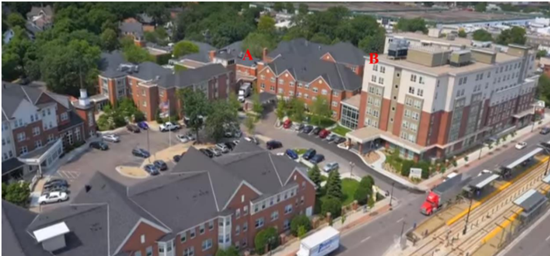
Figure 3. The bird view of the whole facility in 2018. Source from Episcopal Homes Website ( www.episcopalhomes.org )
