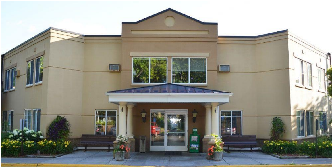
Figure 14. Building facade of Building C in long-term care facility B
