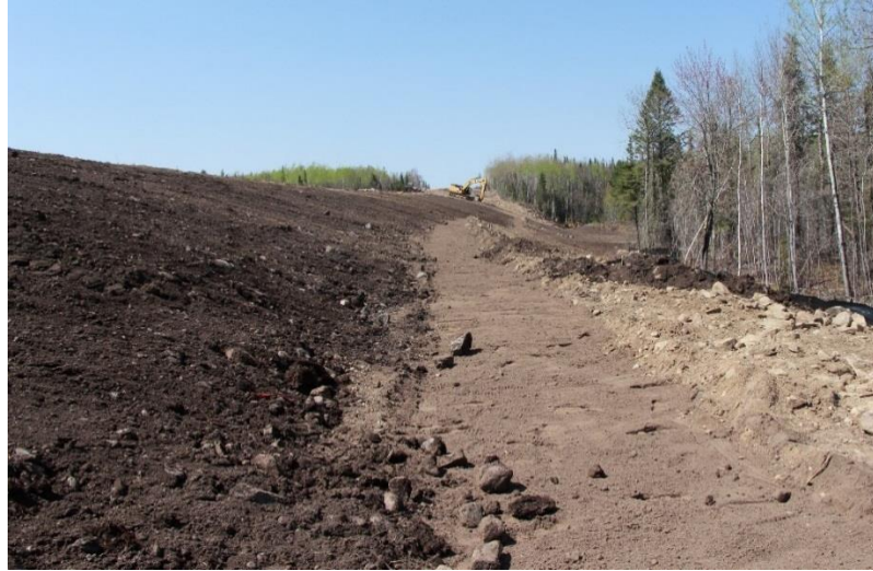
Figure 59. Bioswale construction at midpoint of hillside.
