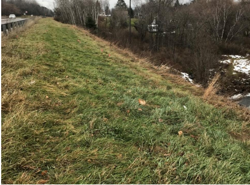
Figure 38. Ground view of the biofilter located over Keene Creek in Duluth, Minnesota.
