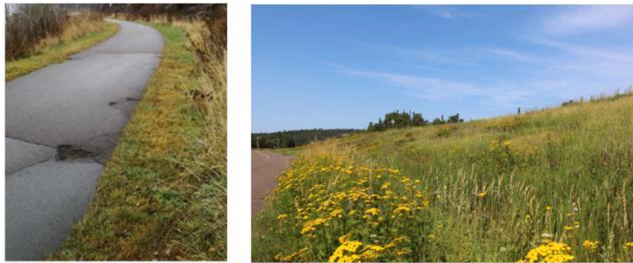
Figure 44. Biofilter along trail (left) and at the south trail access point (right) at the Silver Creek Cliff Tunnel.
