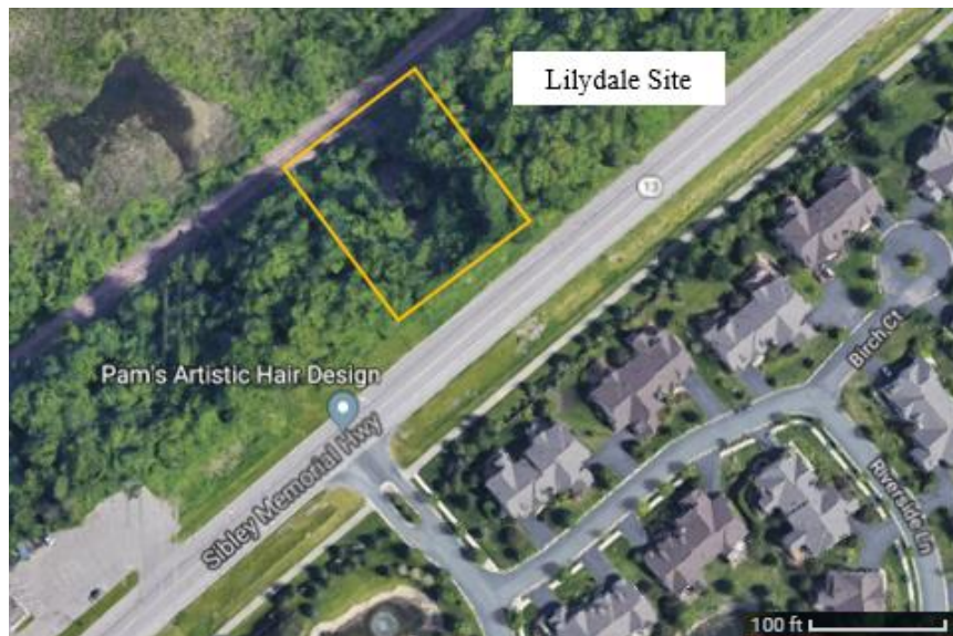
Figure 40. Aerial view of the biofilter located along the Sibley Memorial Highway in Lilydale, Minnesota.
