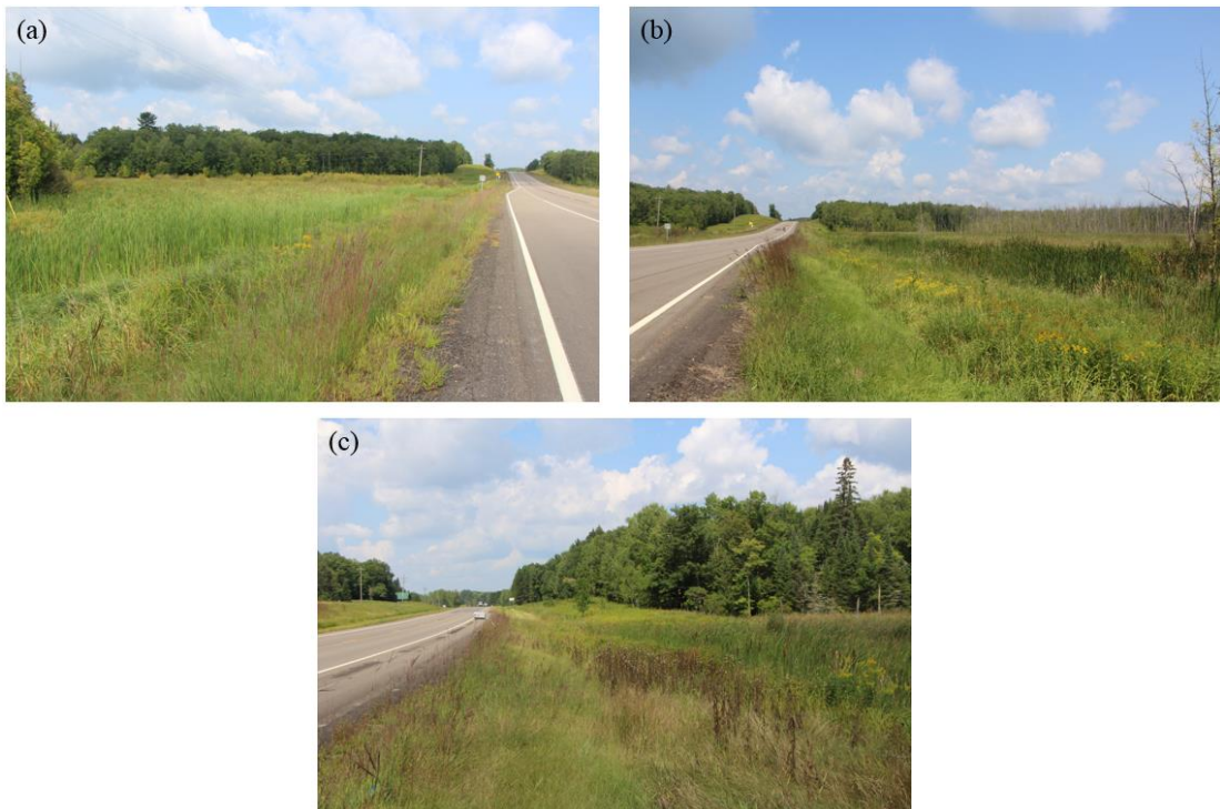
Figure 29. (a) West portion of Crosby Site 1. (b) East portion of Crosby Site 1. (c) Crosby Site 2.
