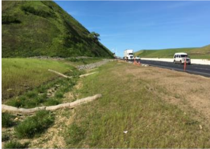
Figure 16. Vegetated swale with temporary check dam along a California highway (Caltrans, 2017).
