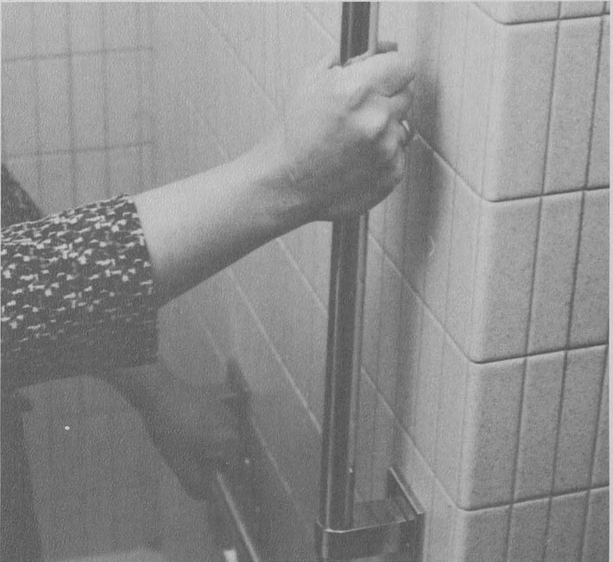
Grab bars must be reinforced and bolted to wall studs to hold a person's weight.
