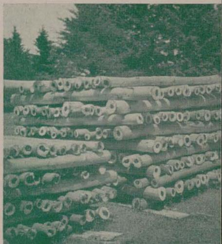
Preparations for treatment—Peel off both outer and inner bark of posts to get good penetration of penta. Stack posts crib-fashion for proper air drying before treatment.
