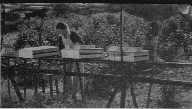
A TEMPORARY BERRY SHED
