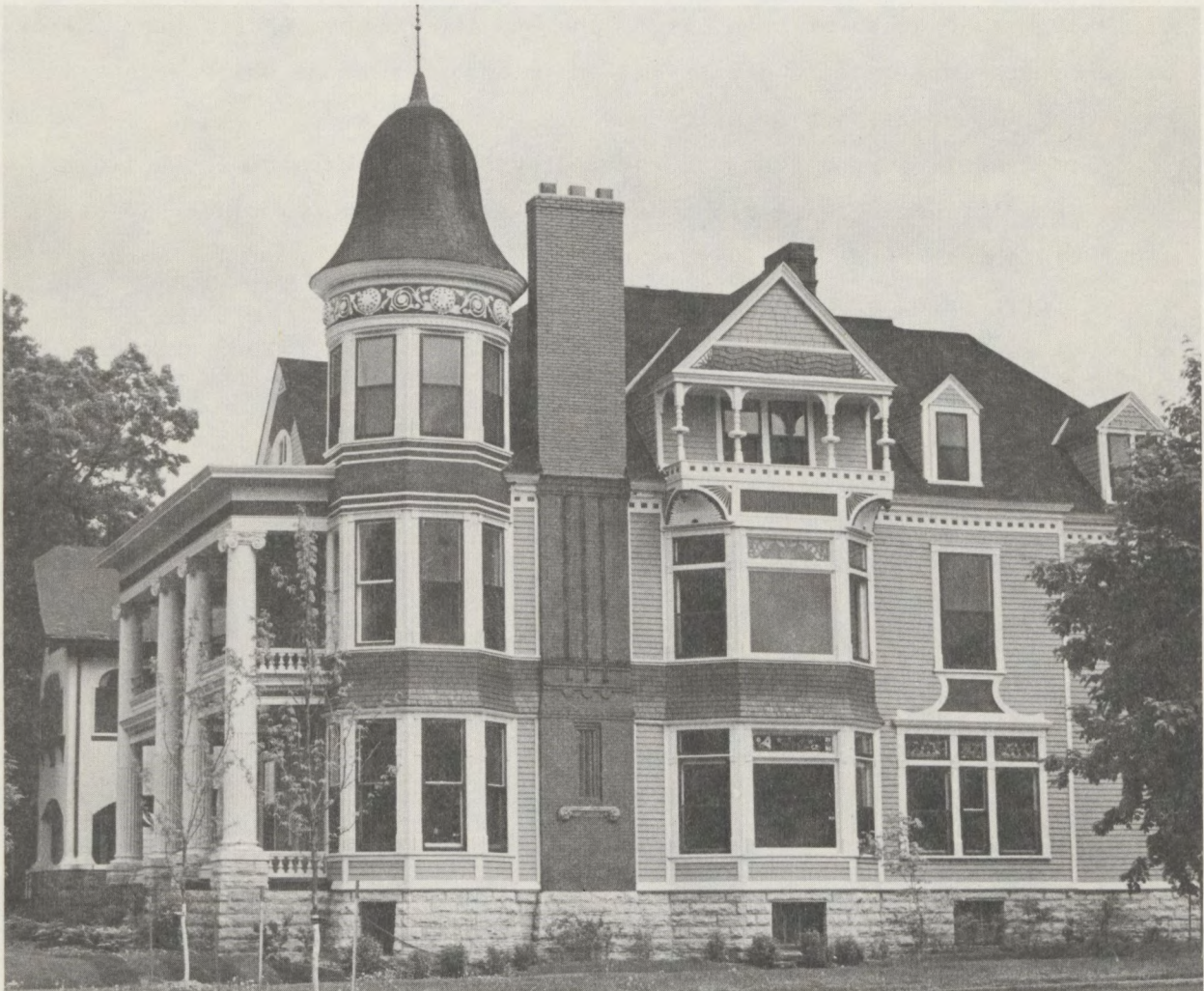
A Building Comparable to Project A in the Historic Hill Area of St. Paul
