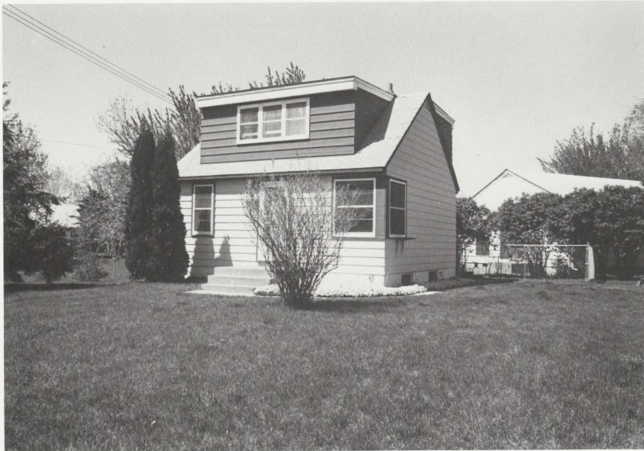
Figure 25. Living space in the attic is expanded by adding dormers.
