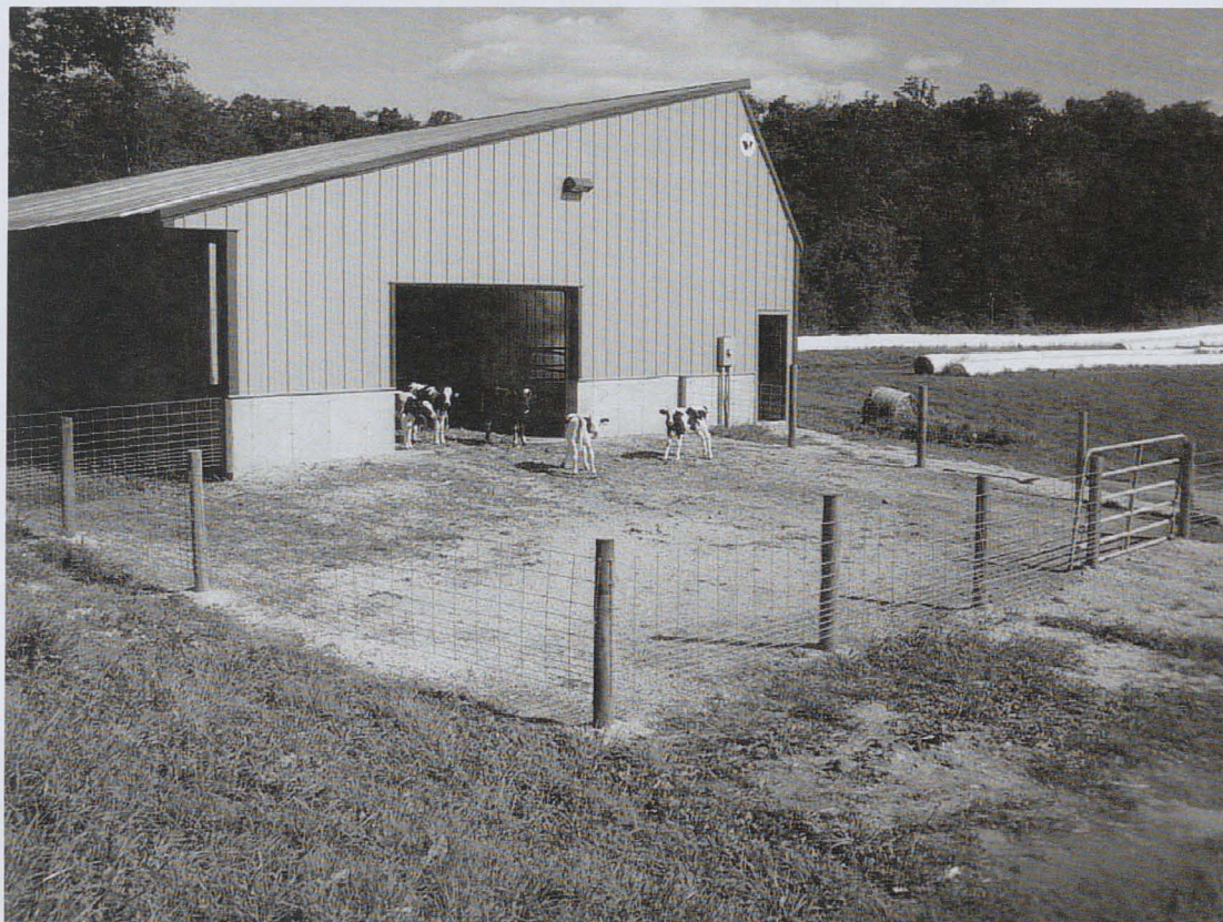
Figure 2. Recently installed outdoor exercise area.
