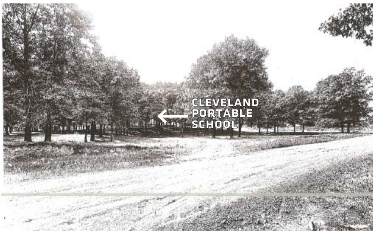
NATIVE LANDSCAPE: THIS PICTURE OF THE PORTABLE SCHOOL THROUGH THE TREES (1916-27) SHOWS THE NATIVE OAK SAVANNA LANDSCAPE PRIOR TO THE CONSTRUCTION OF HOUSING OR PAVED ROADS.
