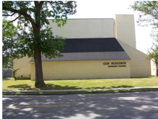
Photo 10: Our Redeemer Lutheran Church as seen from across 28 th Avenue South. Photo taken by Daniel Allen.
