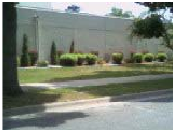
Photo 11: The Qwest building located at 3301 24 th Avenue South in Minneapolis. Landscaping was done recently in an effort to deter graffiti. Photo taken by Bob Kambeitz.
