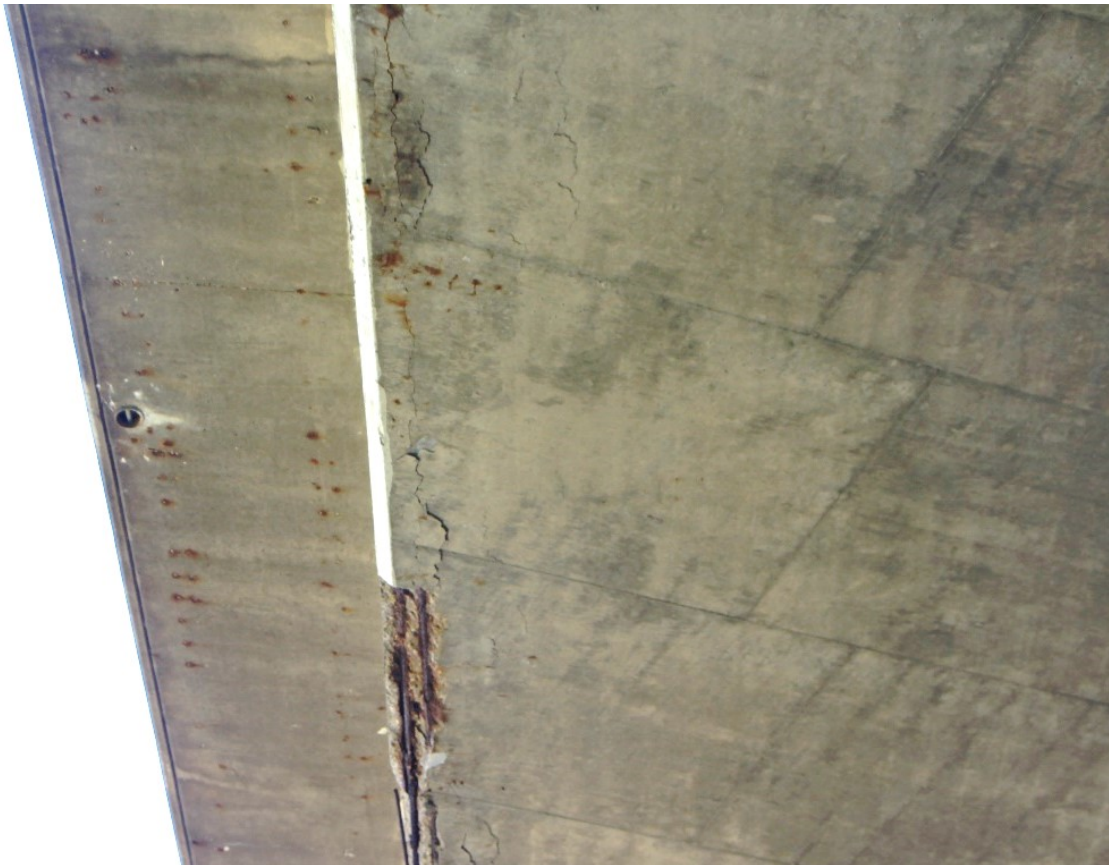
Figure 2.7 Representative image for advanced delamination
