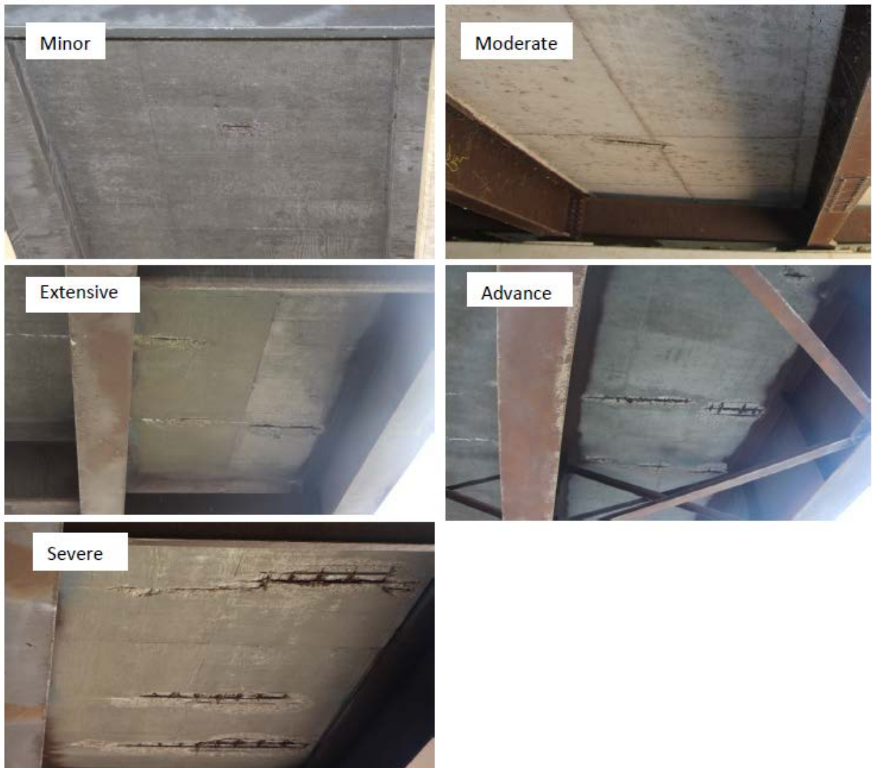
Figure 2.6 Representative images of each category of spalling with exposed rebar
