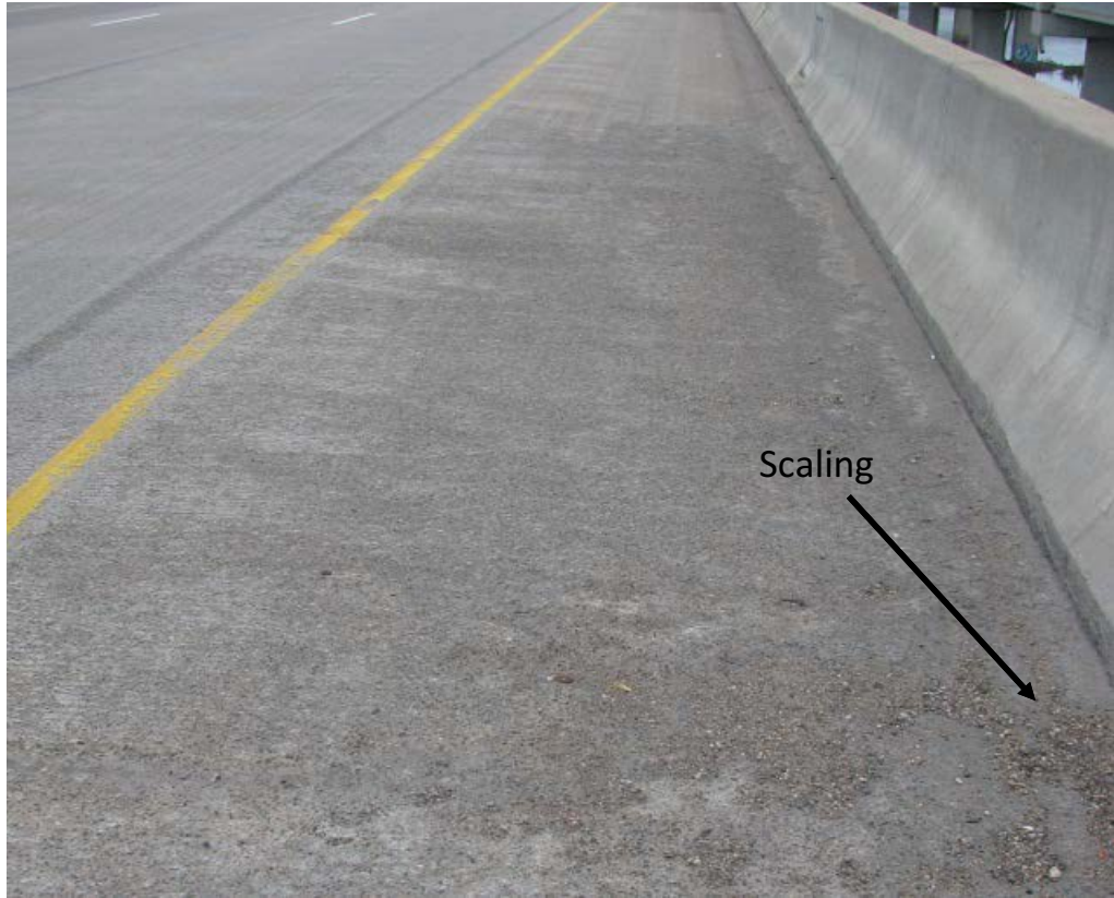
Figure 1.4 Scaling of concrete on the top of the deck (MnDOT, 2017)
