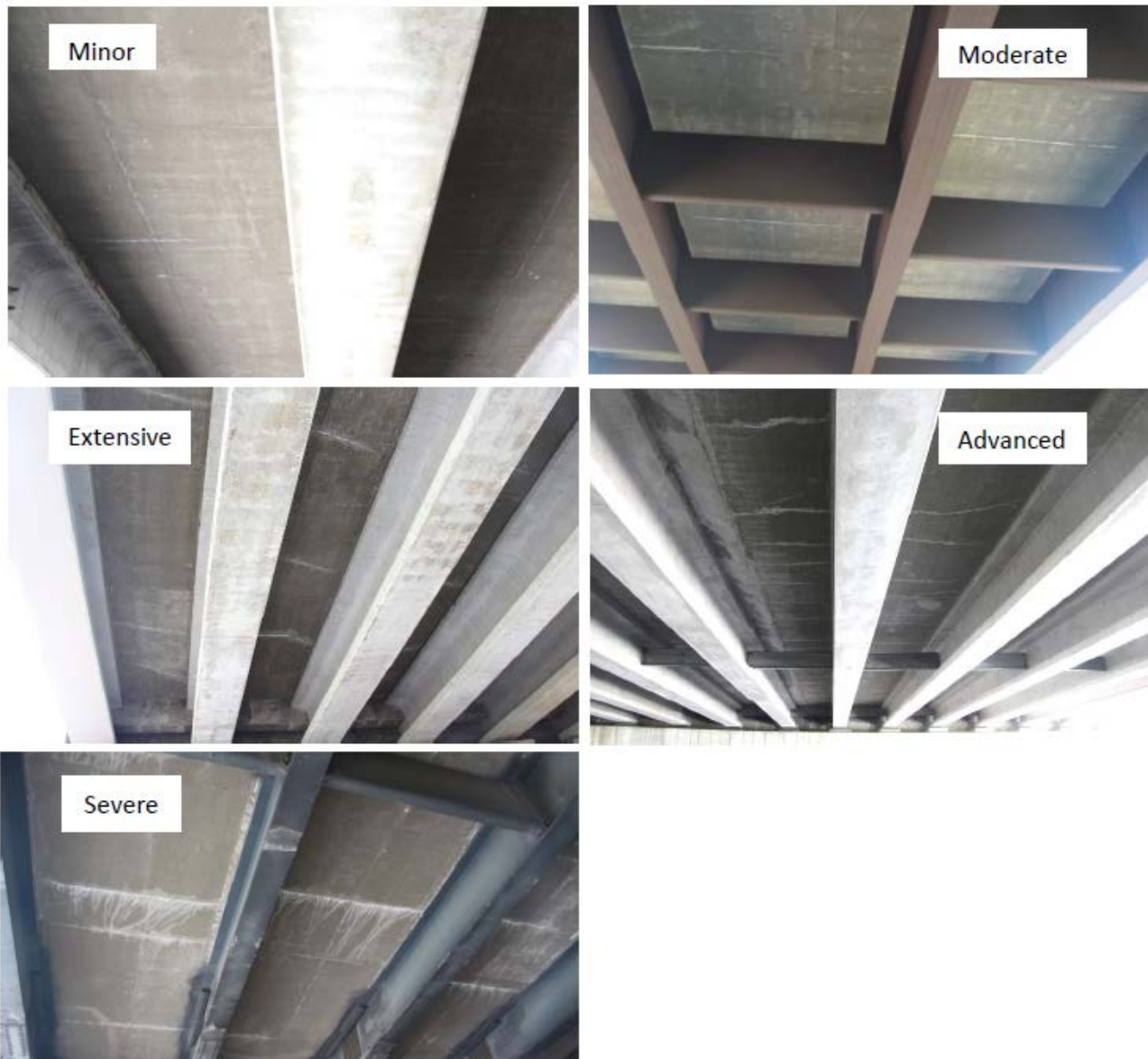
Figure 2.5 Representative images for each category of cracking with efflorescence
