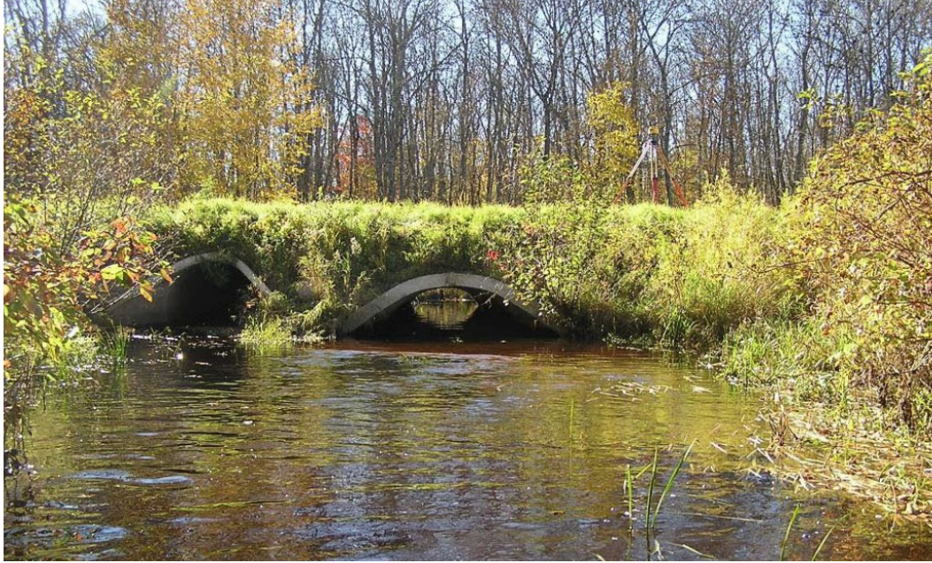
Figure 5.5.13. Existing Moody Creek culverts (Hansen et al. 2011)
