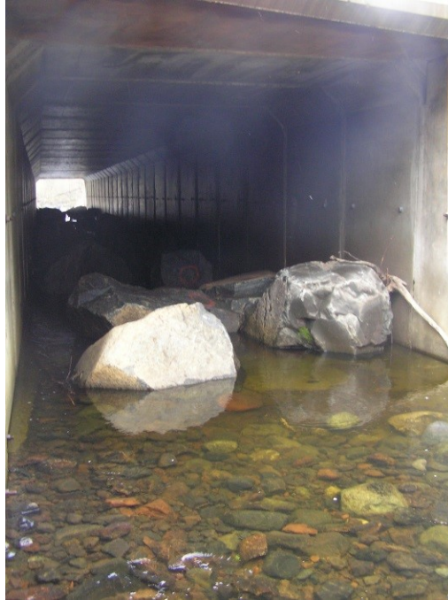
Figure 5.4.2. Boulders added to this culvert are much larger than the apparent bed material, and occupy a significant fraction of the cross sectional area (photo B. Hansen)
