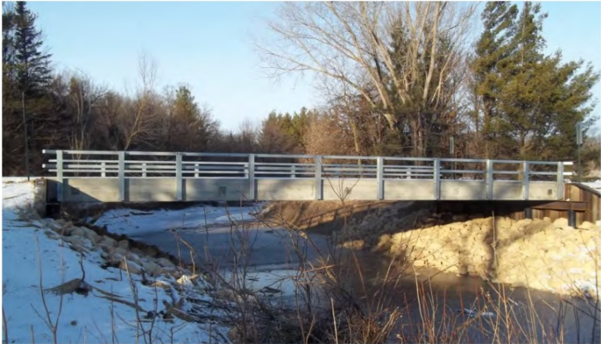
Figure 5.2.1. Side-by-side precast box beams with sheet pile abutments, Blue Earth County Bridge 07547. (Chris Werner presentation CTS, http://www.cts.umn.edu/sites/default/files/files/sessions/17werner.pdf )
