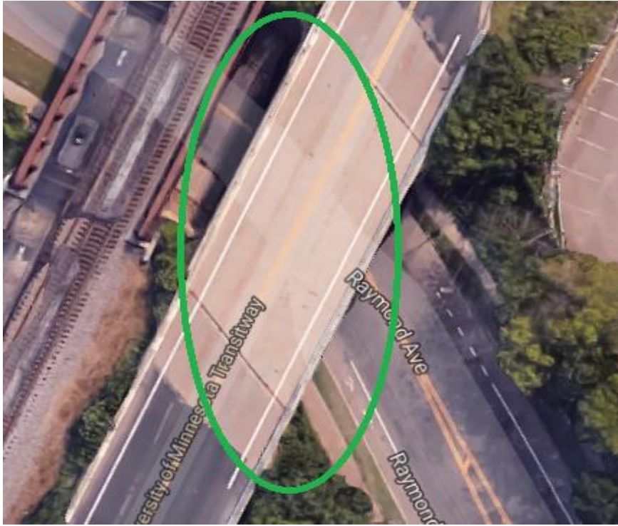
Figure 9.3: Aerial view showing the second candidate bridge and its vicinity (Source: Google Maps)
