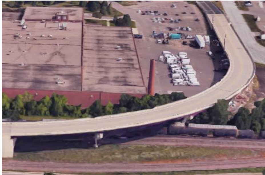
Figure 9.6: Elevation of the third candidate bridge (Source: Google Maps)
