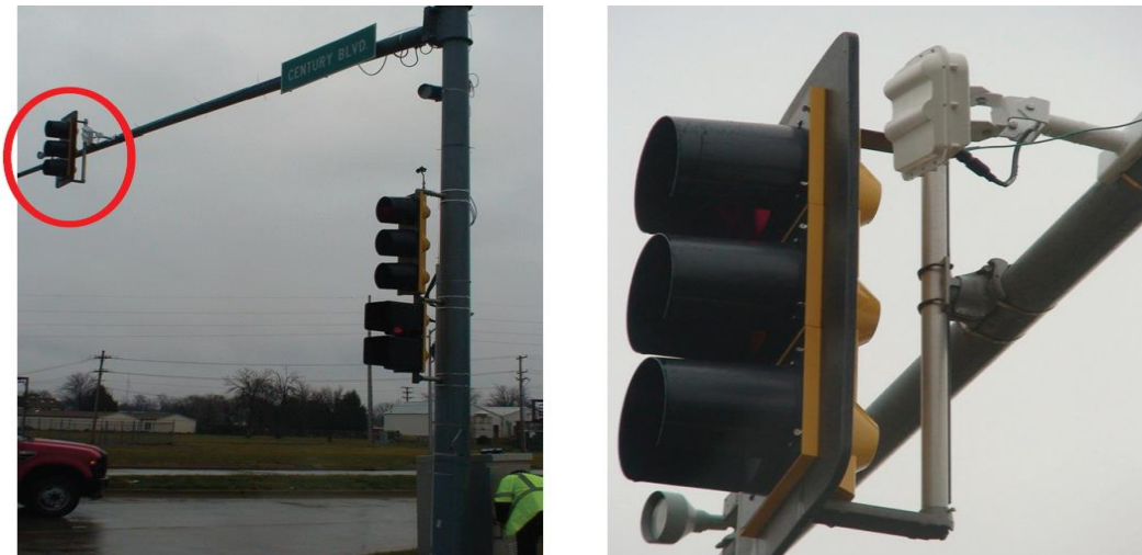
Figure 5.1: Wavetronix radar sensor mounted in doppler mode
