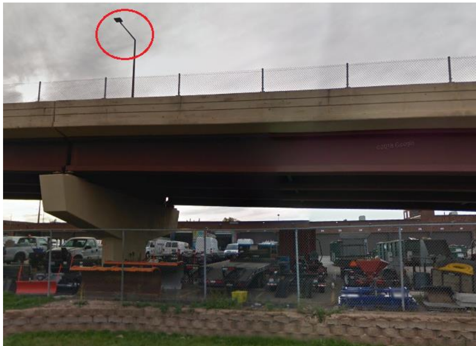
Figure 9.7: Elevation showing the suitable location for strain gauge and radar sensor installation (Source: Google Maps)
