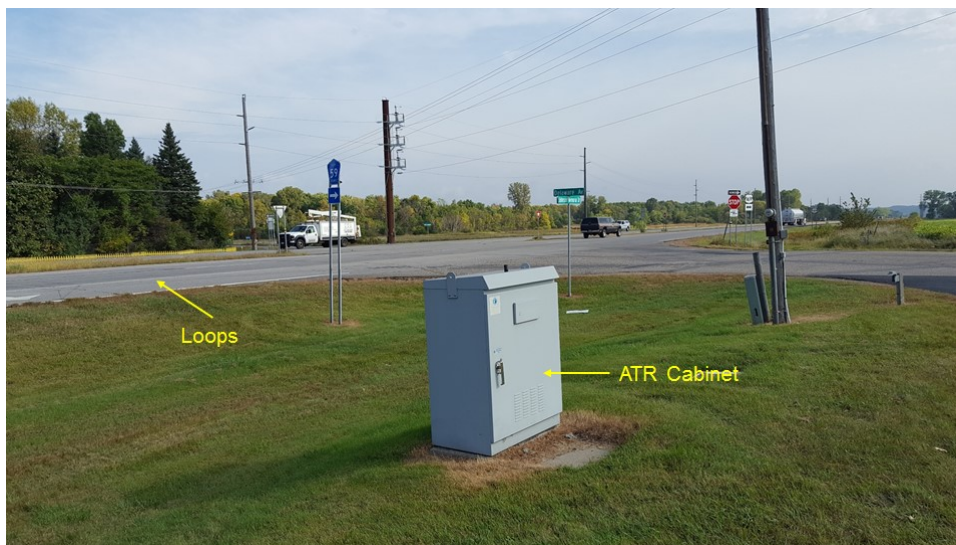
Figure 2.3 Photo of ATR353 Cabinet and Loop Detector Location.
