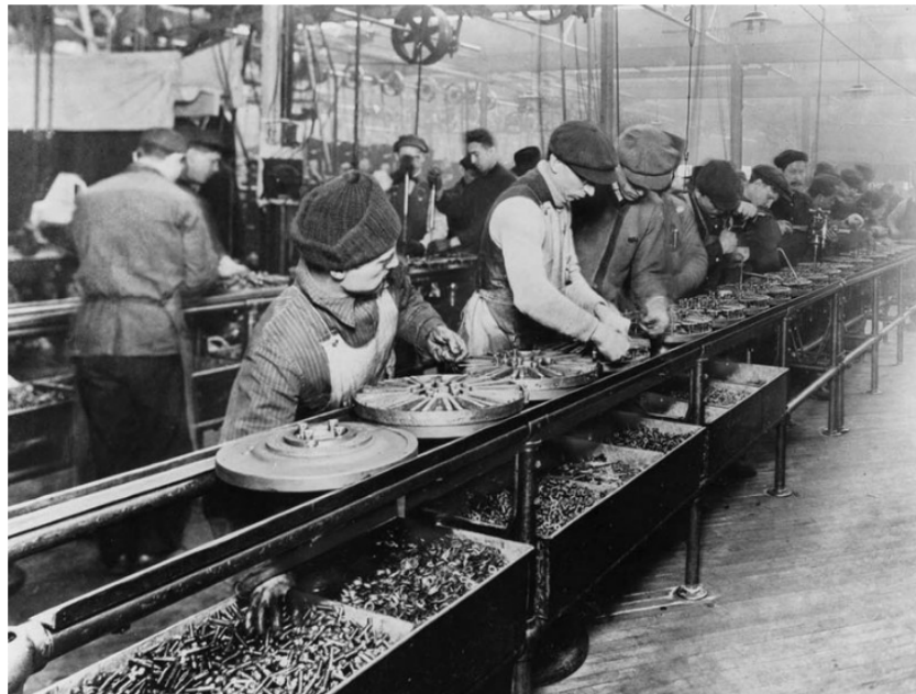
Figure 4. Henry Ford Assembly line in 1913
