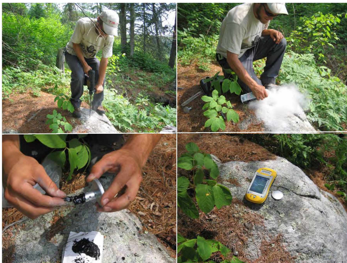
Clockwise from upper left: drilling a hole into the bedrock, using canned air to blow dust from hole, reference mark in bedrock next to GPS unit, applying epoxy to reference mark.
