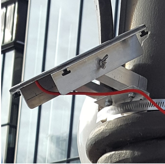
Figure B.4 Solar Panel Mounting Assembly
