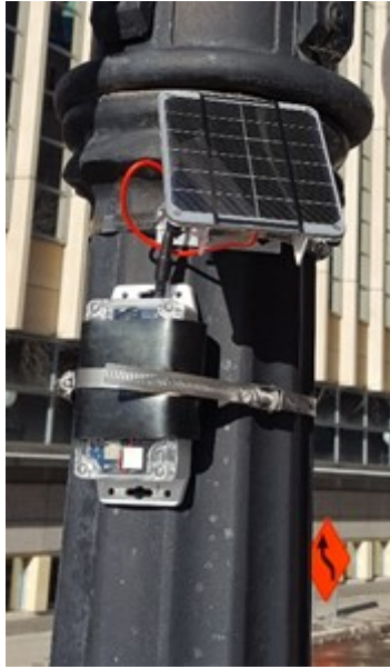
Figure 4.3 Solar-powered BLE on a street light post.
