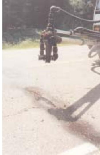
2 *Spray injection patching used on a pothole*
