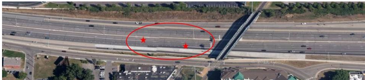
Figure 4.9 Test Site on I-394 in relation to the downstream exit ramp.
