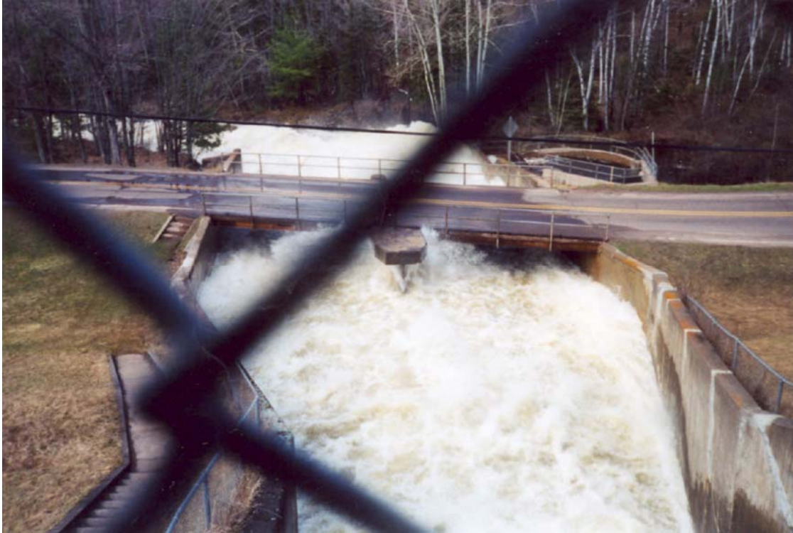
Figure 3.1. A photo of the flood of April 19, 2002 through the channel downstream of the spillway and the bridge.
