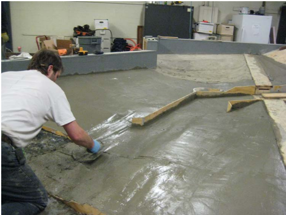
Figure 2.10. The topography of the stream channel and its floodplain was built using formed concrete.
