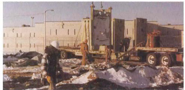
Prairie Correctional Facility Under Construction
