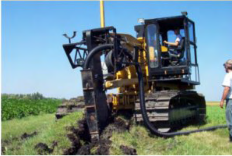
Installing the main tile at the research site.
