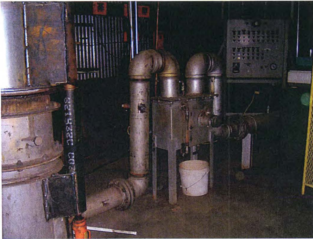
Figure 3 Original Exhaust Piping with Water Quench Tank
