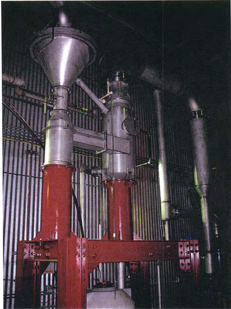
Figure 7 Gas Scrubbing and Exhaust Piping
