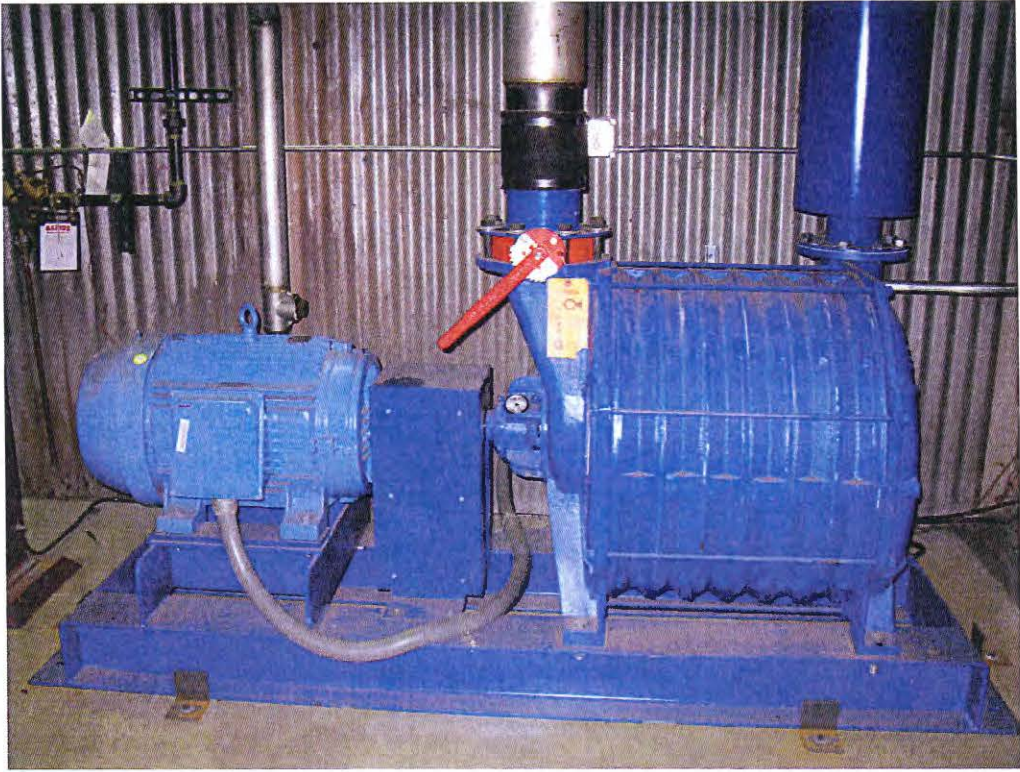
Figure 8 New Exhaust Blower
