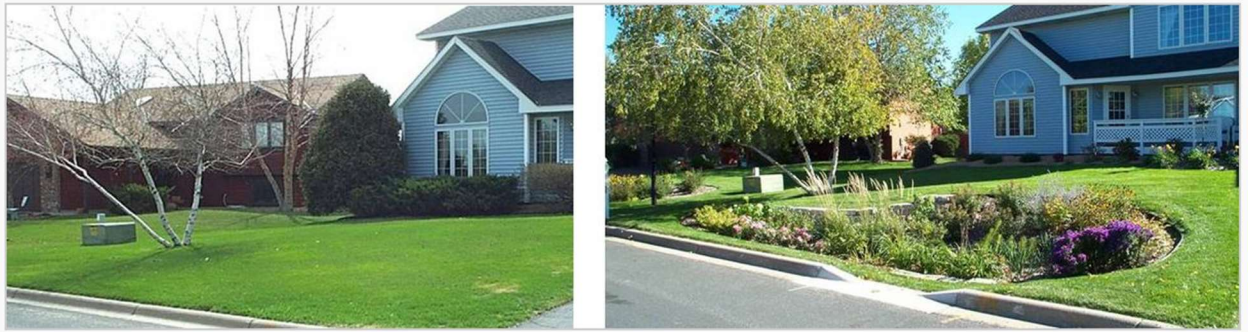
Figure 3A. Before and after photos of a rain garden project in Burnsville, MN. Notice the curb cut in the forefront of the picture on the right, this allows for capture of water during a storm event. Once the garden is at maximum capacity, water will bypass the garden and continue to flow down the curbside to either the next garden or into the stormwater network (Minnesota Pollution Control Agency 2016).
