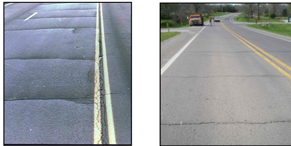
Figure 3: Transverse cracking of asphalt pavements
